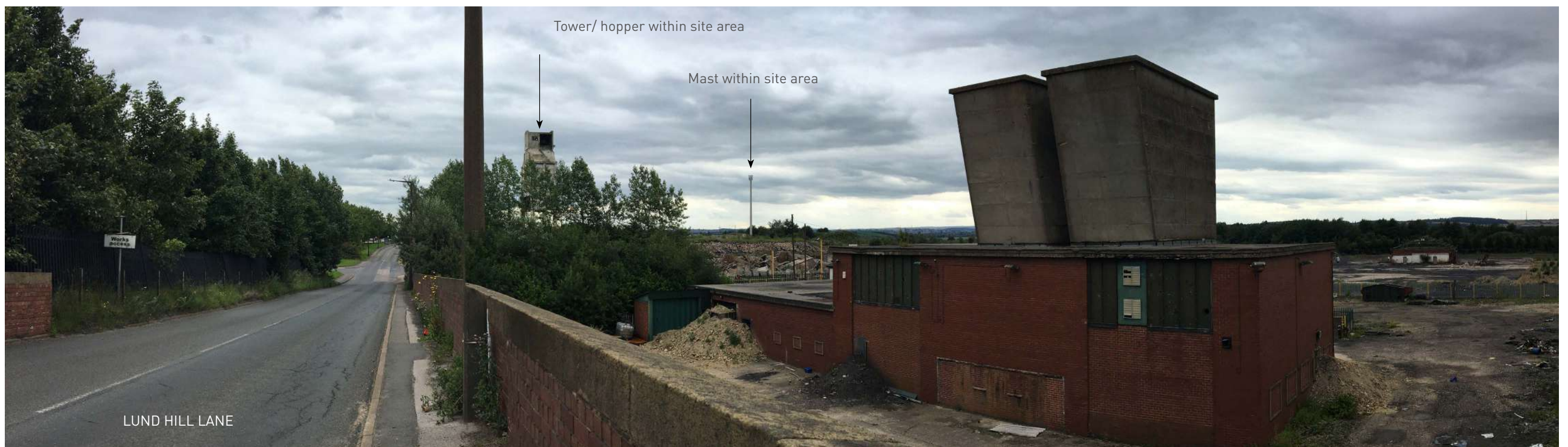
Photograph 10: From bridge on Lund Hill Lane looking south west
