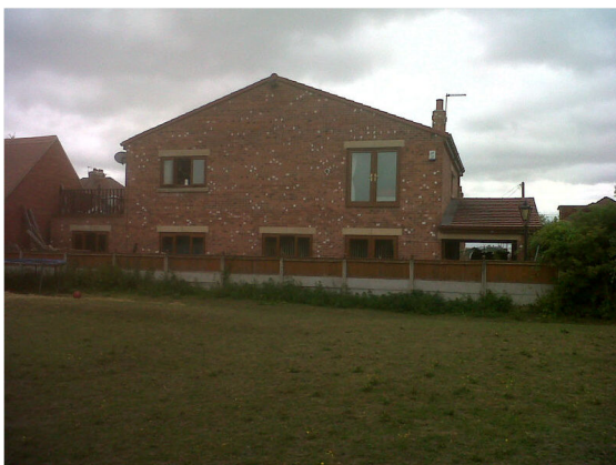
Figure 2 Rear Elevation from the paddock which is in another ownership
