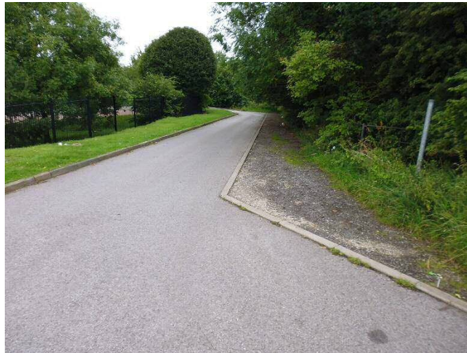
Photo 2: Pedestrian Infrastructure on St Helen's Boulevard (East of Access)
