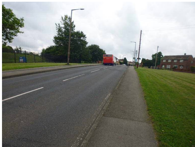
Photo 3: Pedestrian Infrastructure on Carlton Road
