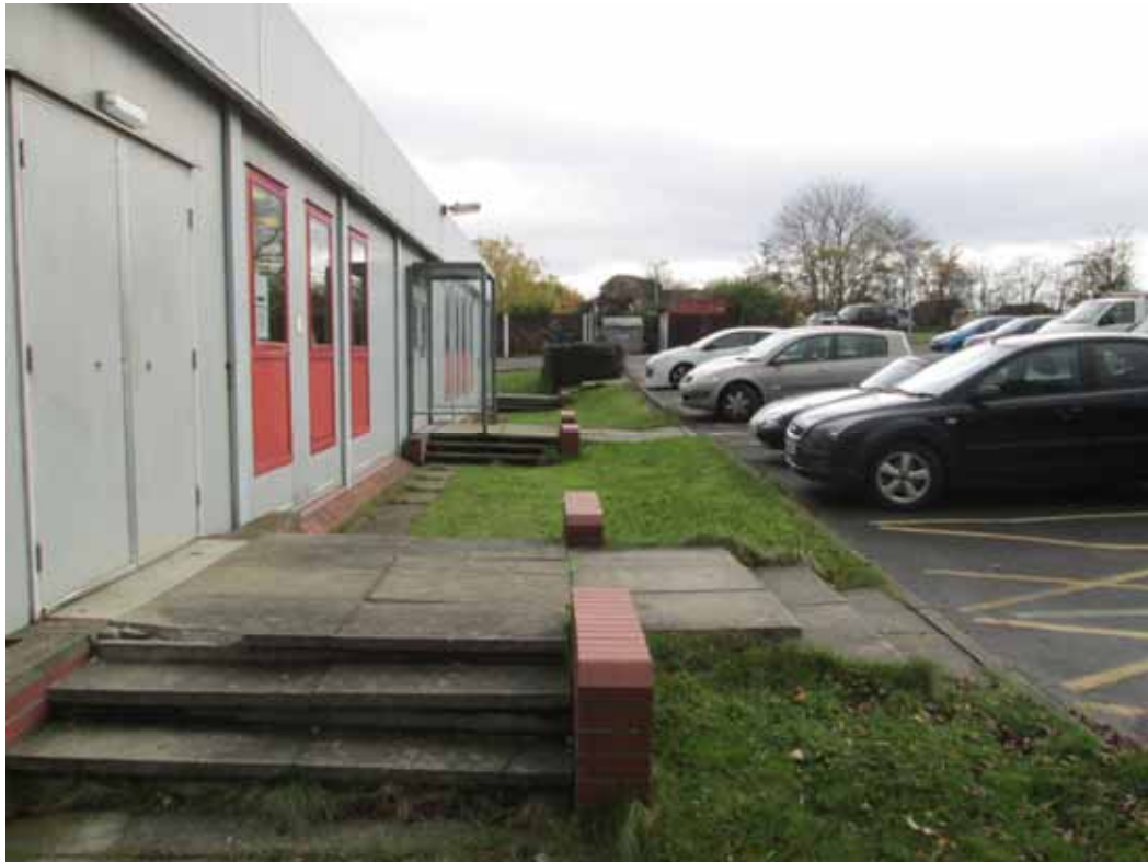
Photo 9 – Steps into building to East
