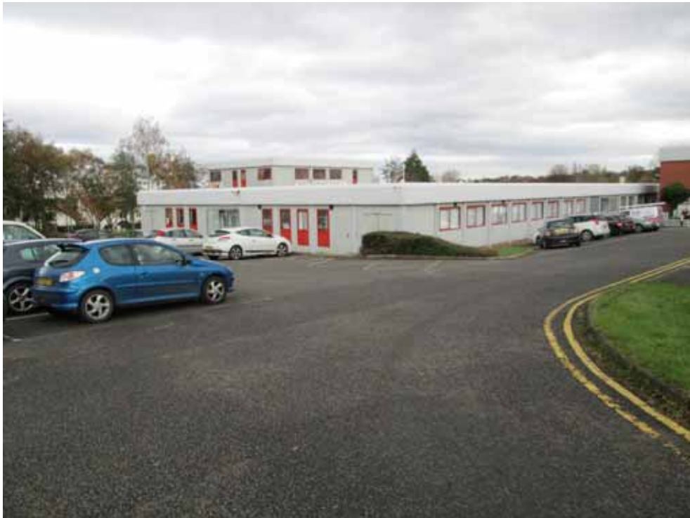
Photo 1 – Existing building to East of site.
