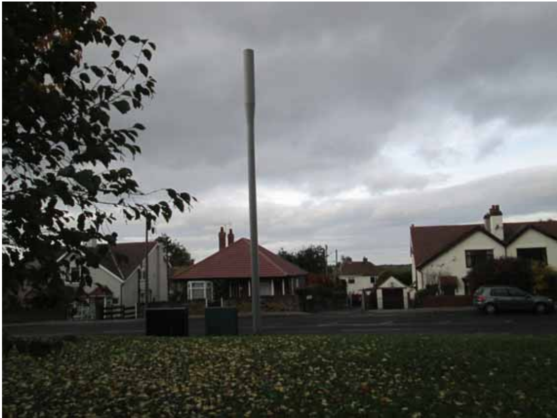
Photo 5 – Mobile telephone mast
