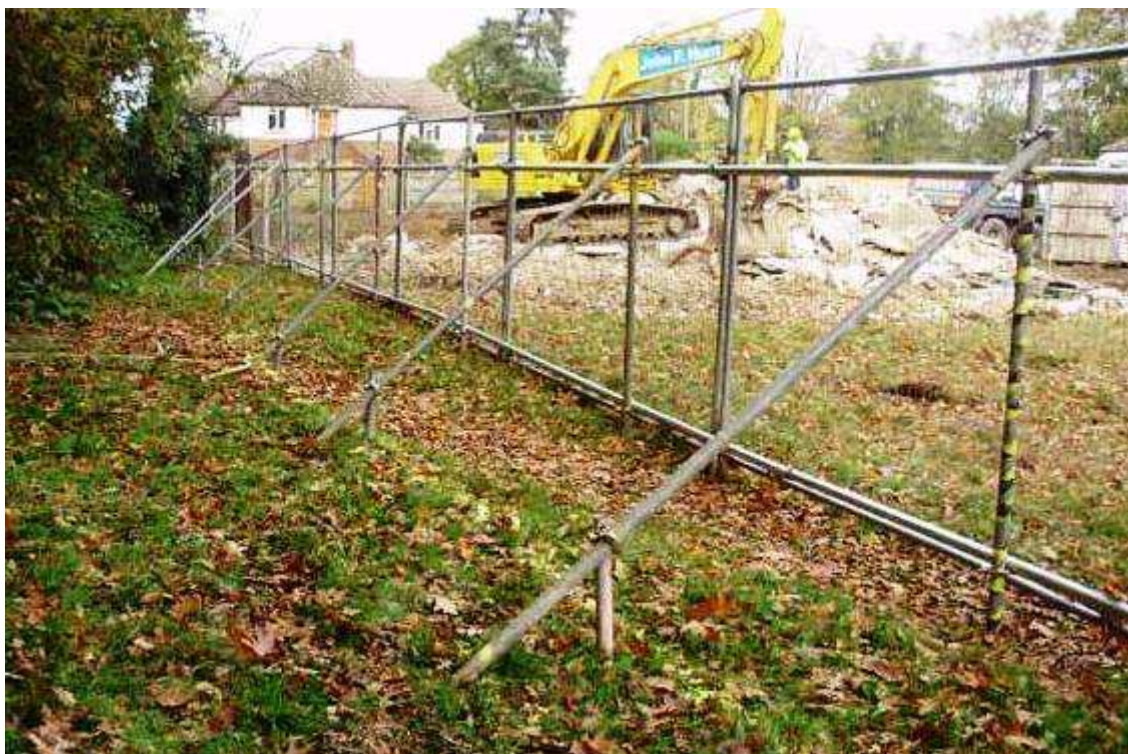
Figure 2: 'Photo of Fencing to BS 5837: 2012'.
