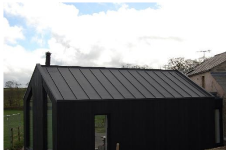
Dark Grey metal standing seam roof Anthracite Grey RAL 7016
