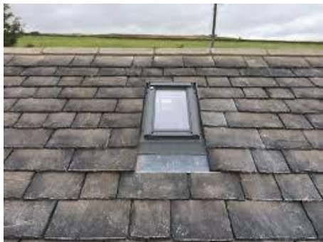
Existing/new Natural Yorkshire Stone Roofing tiles
