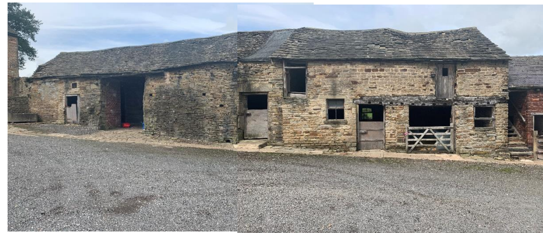
Existing frontage of the barns.
