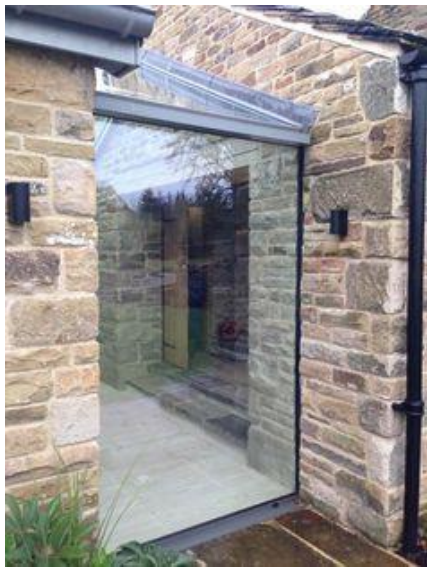
Curtain wall system to form glazed link
