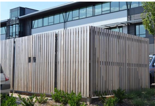
Fuel tank enclosure base with 2.1m high hit and miss fencing panels fixed to precast concrete posts
