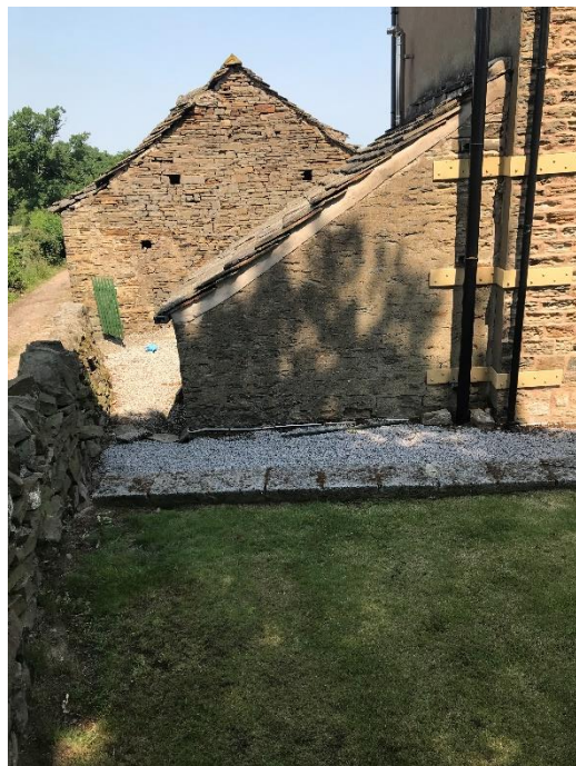
Existing extension between house and barn
