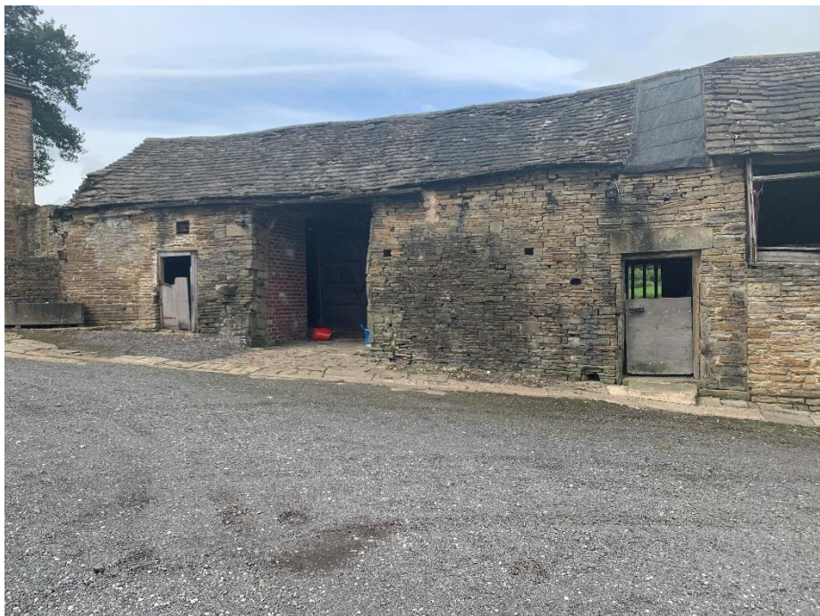
Views of the front of the barns from the property courtyard.
