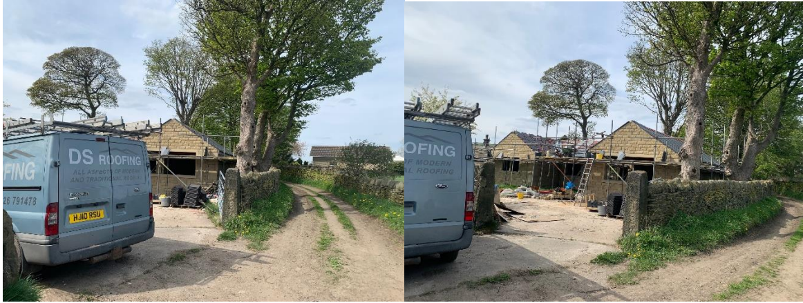
Current site photos April 2022
