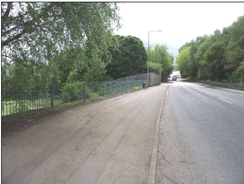
Plate 1: View along Wombwell Road, with the site to the left. Note the drop in height between the road and the site. Looking south-west
