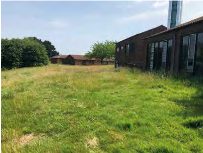
Plate 2 – Boiler Room and chimney (possibly incinerator) at the north of the Site.
