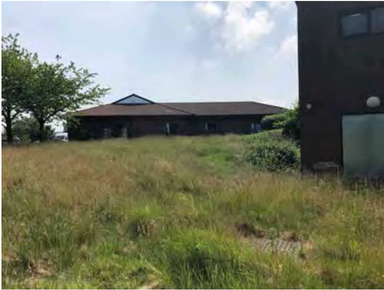
Plate 6 – Dipping site levels and overgrown former grassed areas.
