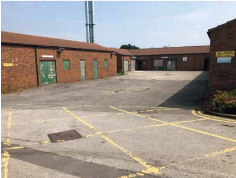
Plate 4 – Disused Area of the Keresforth Medical Centre.
