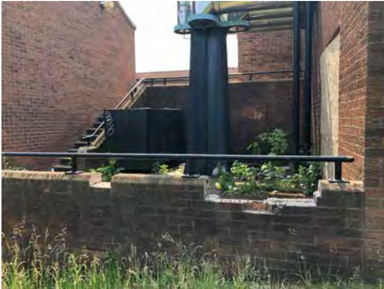
Plate 1 – Rear of Boiler Room, AST in raised area.
