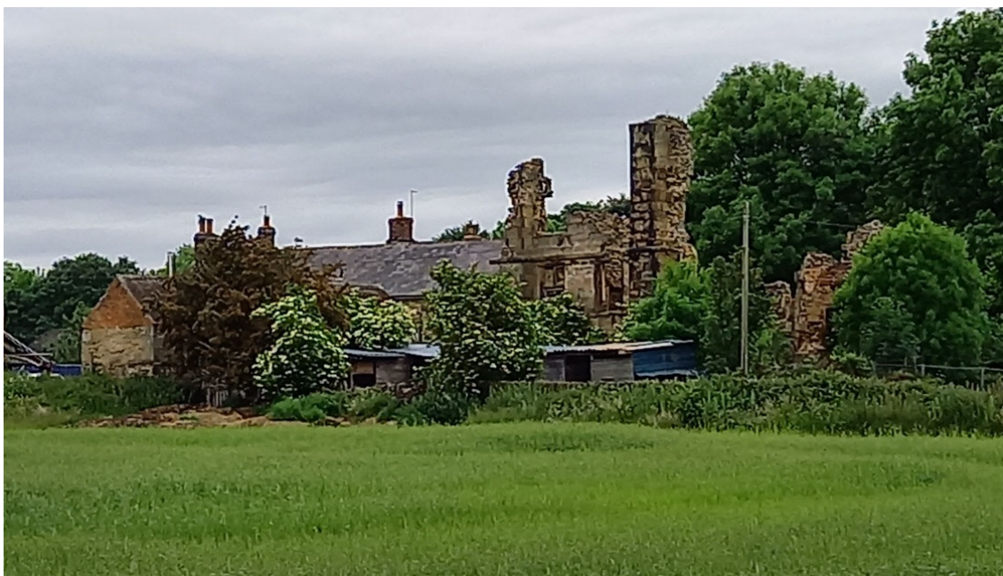
Plate 5: South elevation of Tankersley Old Hall, with stabling in foreground and Old Hall farmhouse behind
