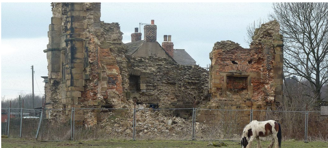
Plate 6: Remaining east elevation of Tankersley Old Hall (Tankersley Parish Council 2013)
