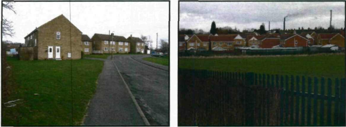
Figure 4 - Buildings located within immediate area
