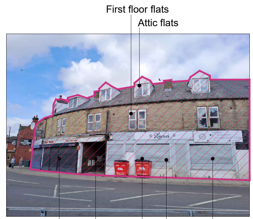
PHOTO 2 Remove and dispose of existing steel roller shutters and housings to all shop fronts including shop windows & entrance doors.
