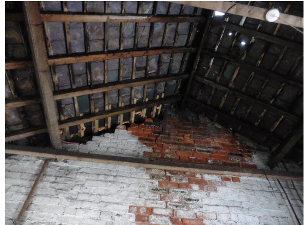
Eastern section open to roof and unlined
