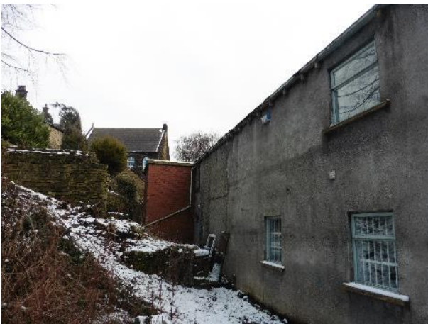
Northern elevation with flat-roofed extension
