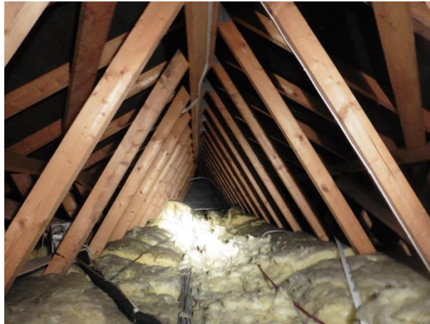
Small, well-sealed roof void
