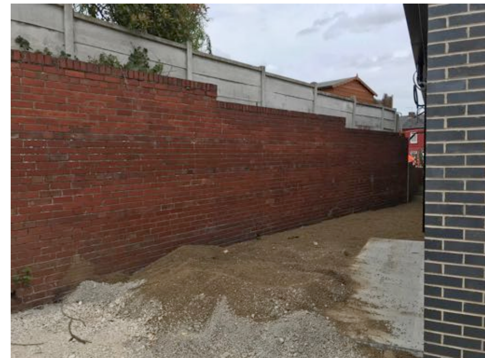
boundary retaining wall & concrete fence
