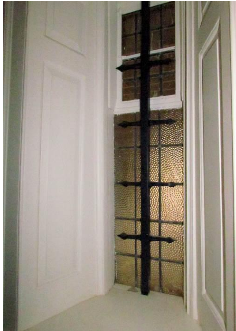
Interior Face of Window
