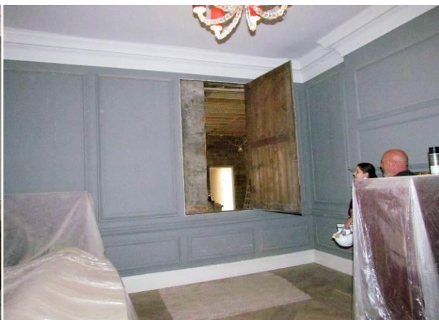
Opening in Panelling
