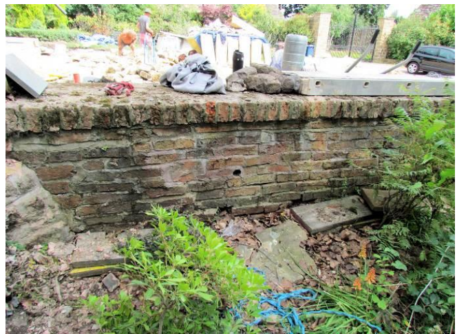
Internal Face of Wall
