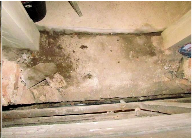
View of Stone Threshold
