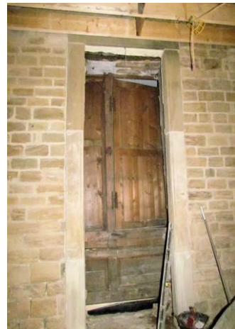
View of Rear Face of Panelling Across Window
