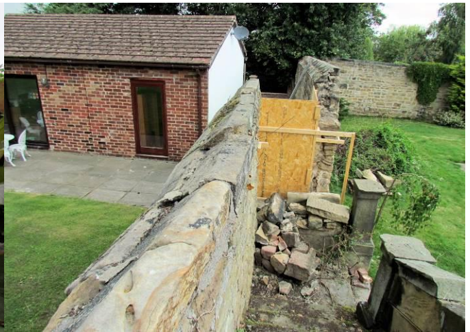
Triangular Coping, West Side
