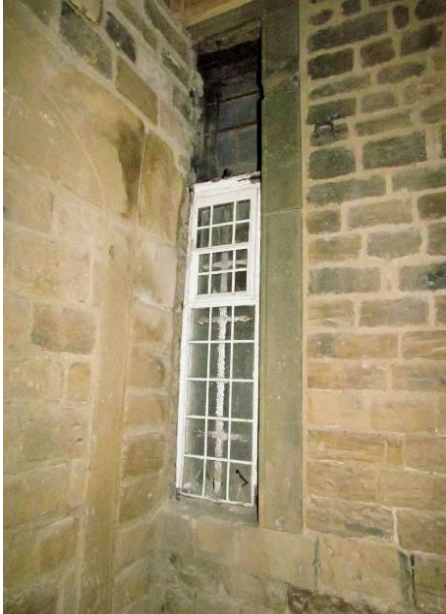
Formerly Exterior Face of Window
