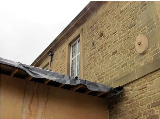
Detail of Cross Window
