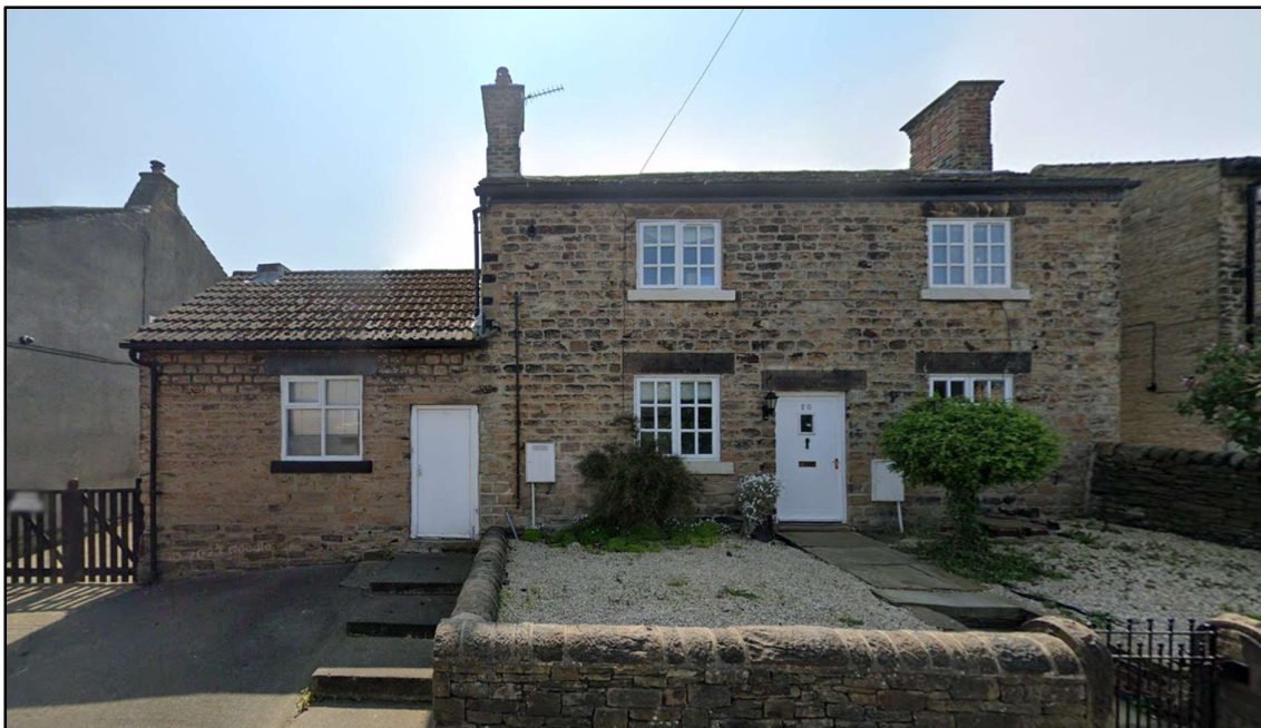
Figure 2 - Photograph of site from Darton Road
