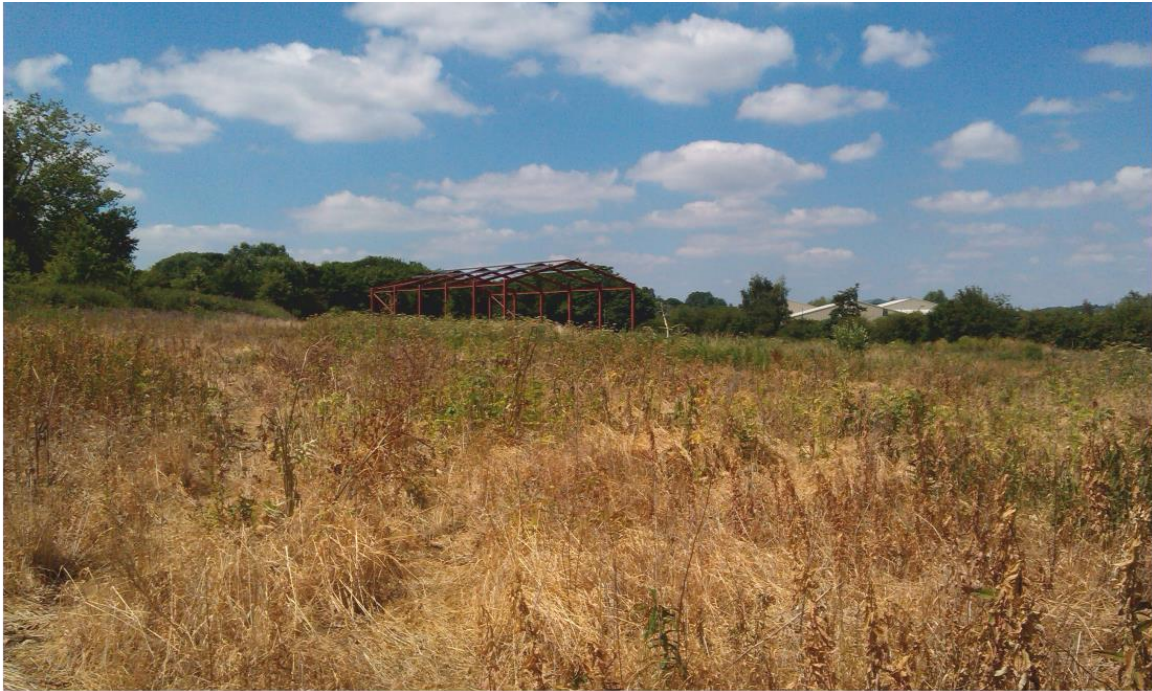
Plate 7 General view across the Site, looking north-west
