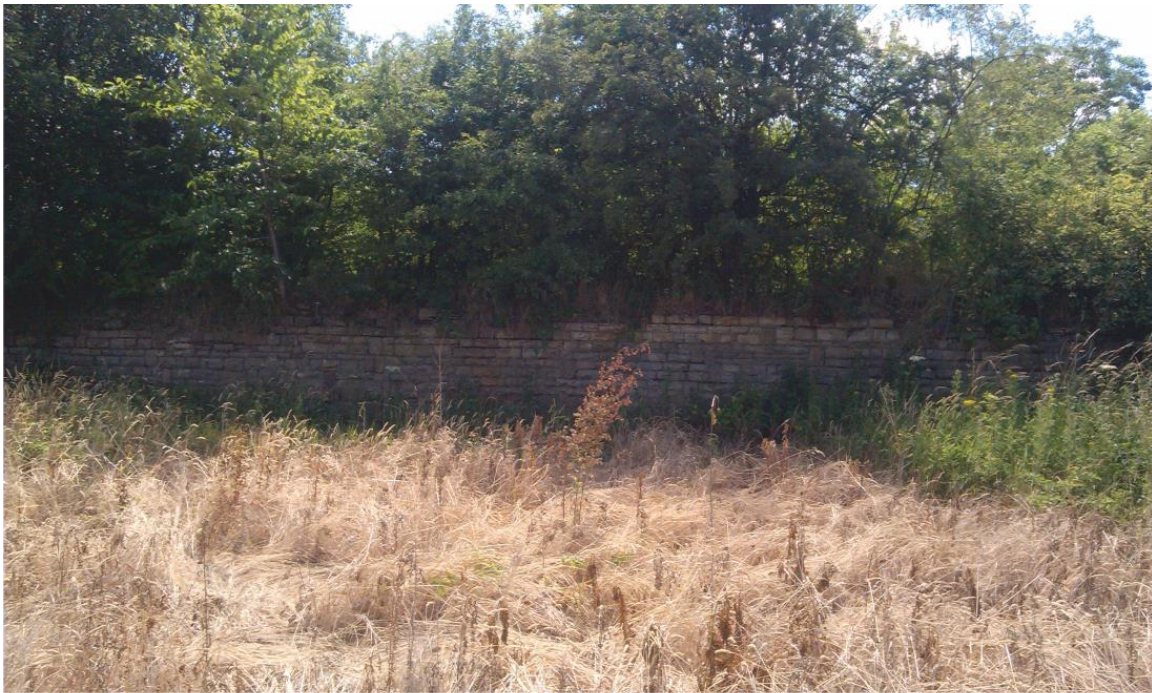
Plate 5 Stone wall at the western end of the canal bank
