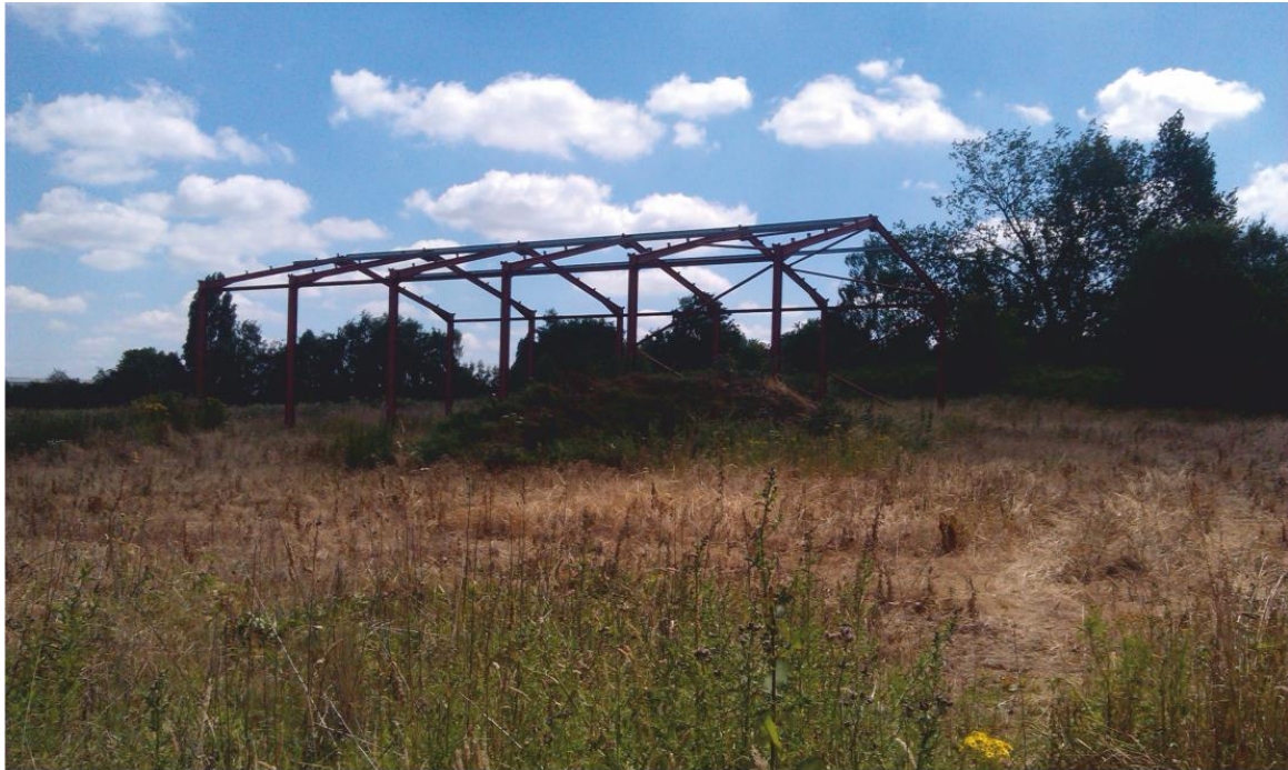
Plate 1 Building structure towards the western extent of the Site, looking south-east
