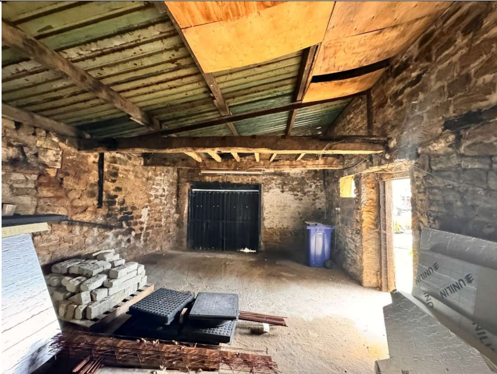
Photo 5: View on internal section of lean to
