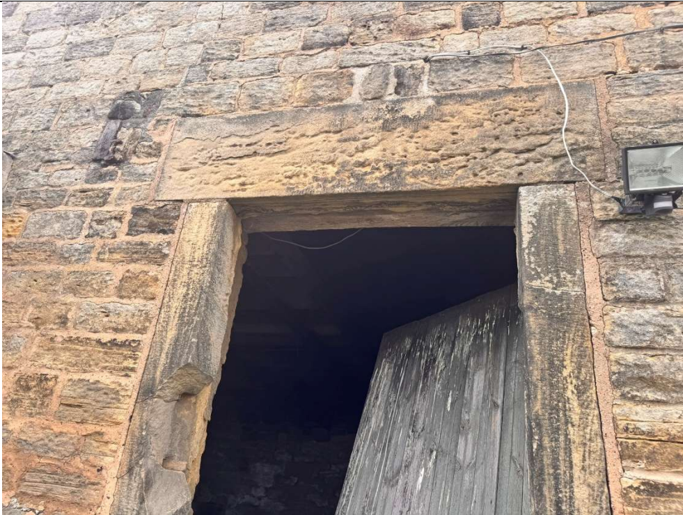
Photo 7: Typical support arrangement around doors/windows
