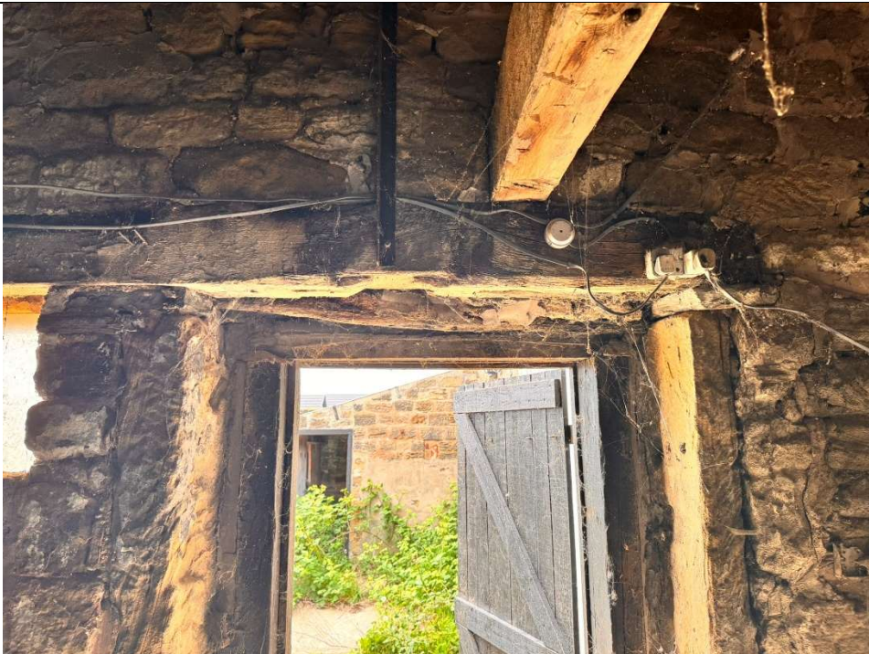
Photo 8: Internal timber lintel
