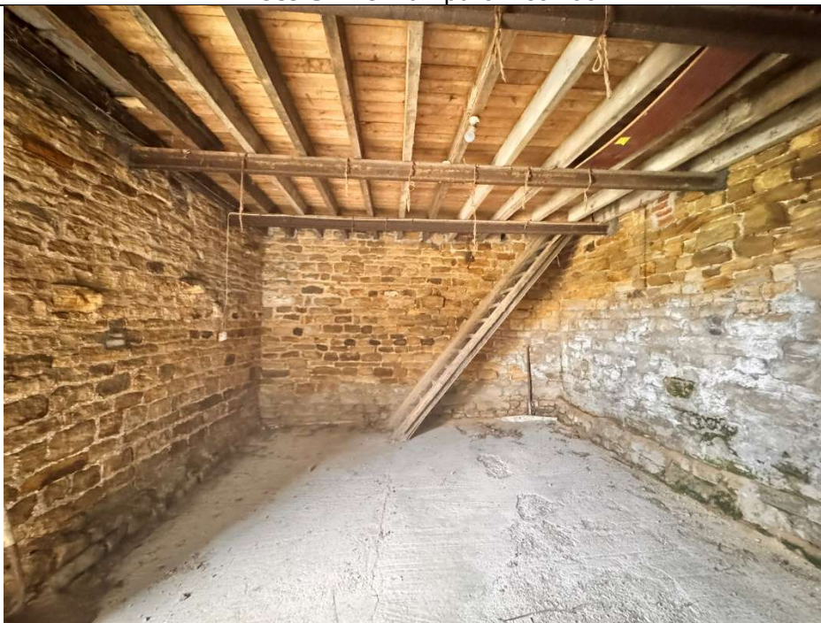
Photo 4: Underside of first floor and concrete ground floor structure
