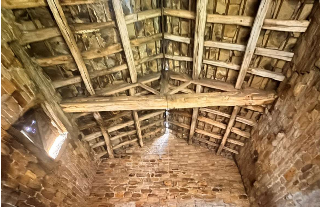
Photo 1: Typical view on underside of roof structure
