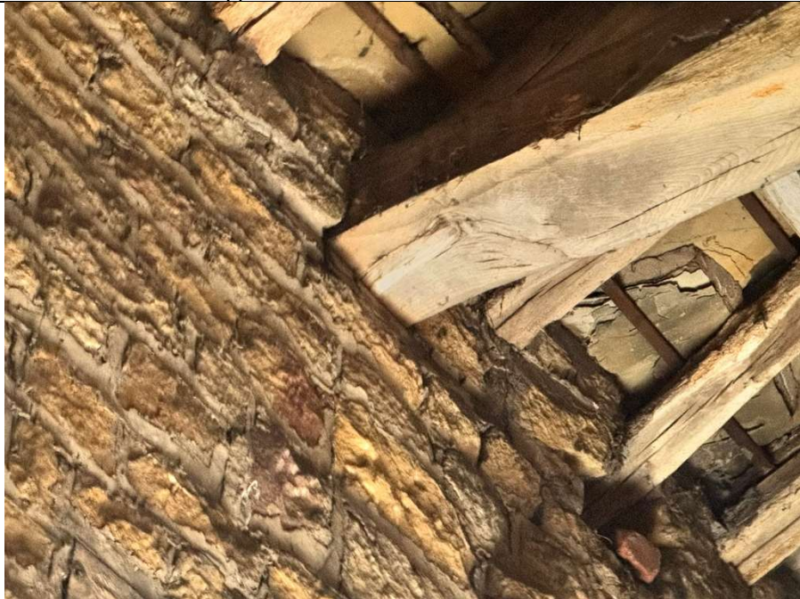
Photo 2: Truss bearing onto external stone wall
