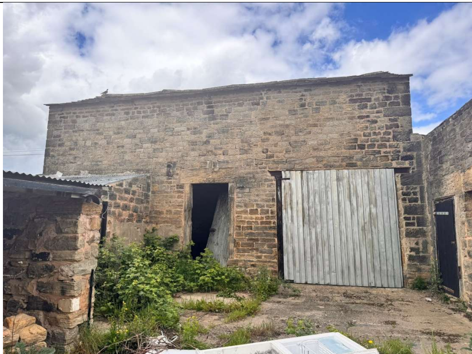
Photo 6: View on main barn elevation, purlin over main door replaced with steel
