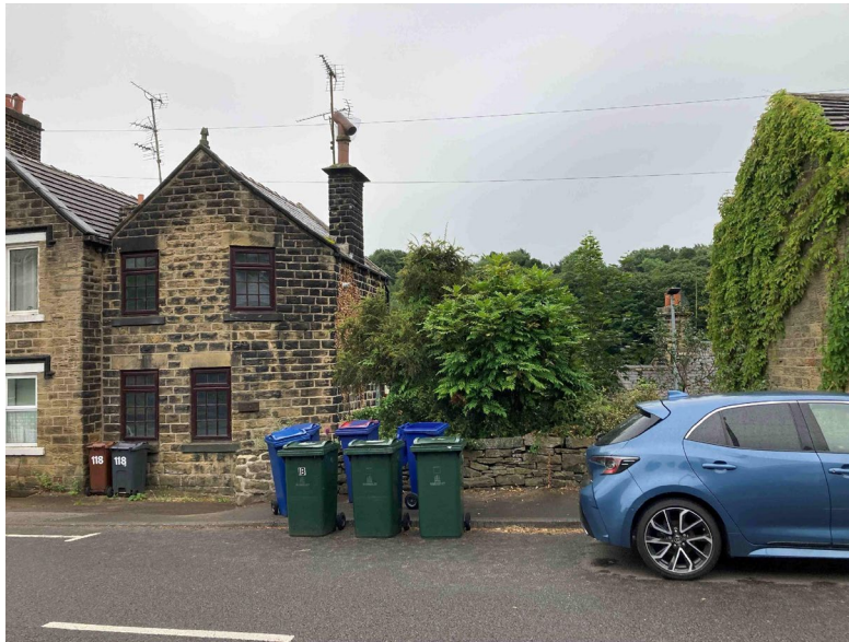
Photograph 1 - No.118 from across Manchester Road. The proposed outbuilding site is directly behind the No. 118 and the trees adjacent. i.e. not visible
