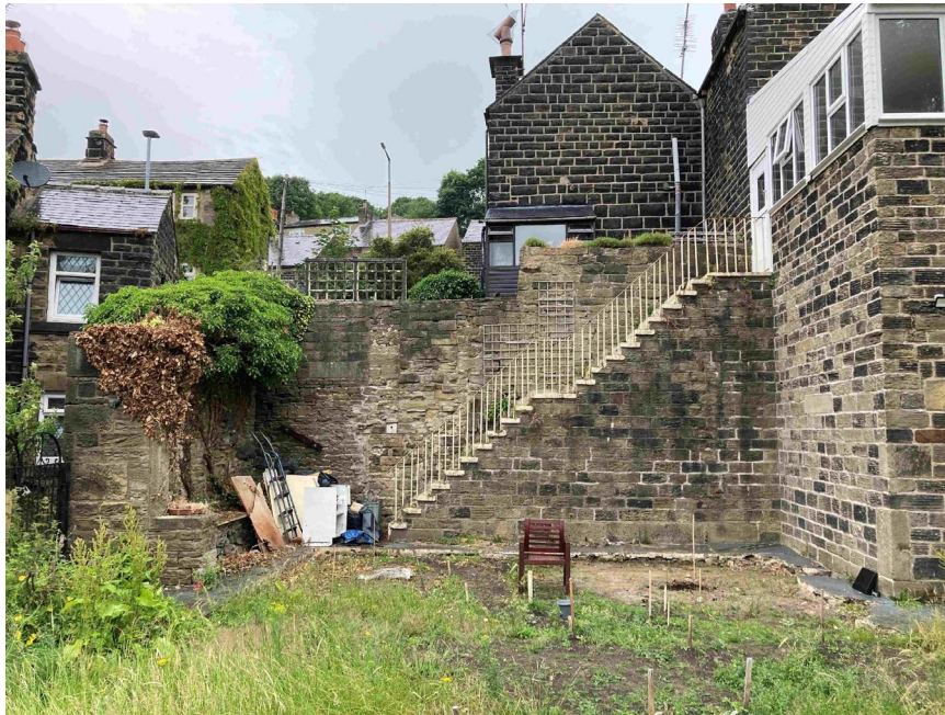
Photograph 5 - A view to the site of the outbuilding from the South boundary. Note the elevated neighbouring property at No.118, and the existing two storey element at the rear of No. 116. The significant boundary wall to the left of the photograph is that to the public footpath.
