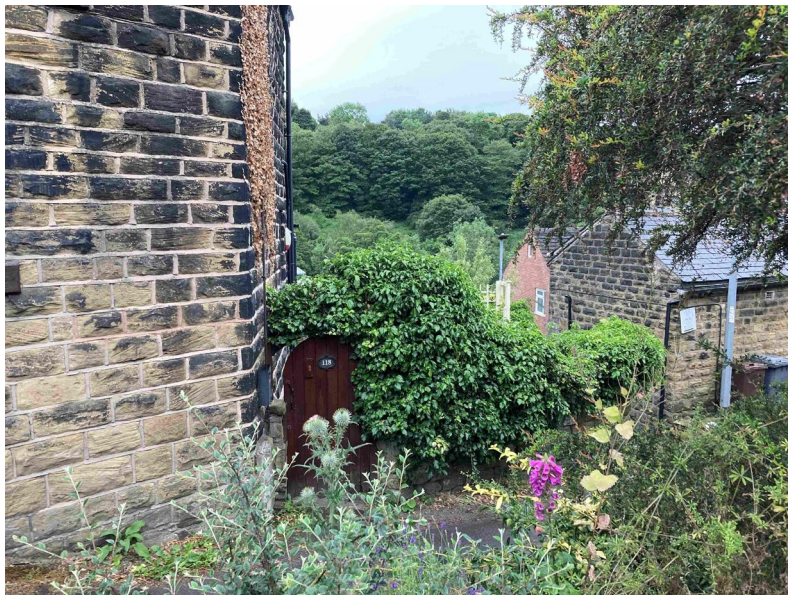
Photograph 2 - No.118 from the entrance of Mill Lane. Again the proposed outbuilding site will be behind the gate and associated planting. i.e. again not visible
