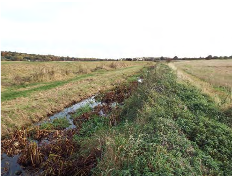
Photograph 4 - Looking east along Bulling Dike as described in TN4. The Wombwell Ings hide can be seen in the distance to the north of the ditch.
