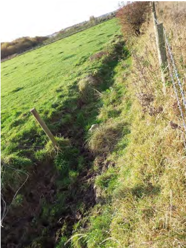
Photograph 10 - Showing the dry ditch just outside of the site, adjacent to the southern boundary as described in TN10.
