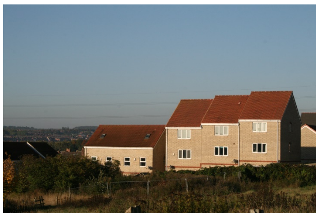
Figure 13 – Verona Rise viewed across the site. This new development was completed in a few years ago and has a range of different house types.
