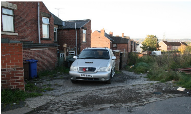
Figure 16 – Rear of the properties on Snape Hill Road. This is the access at the most Easterly point of the site.
