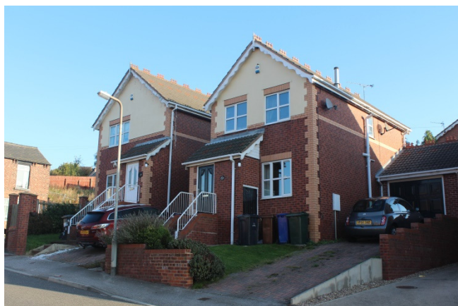
Figure 20 – Examples of houses on The Willows development, across Snape Hill Road.
