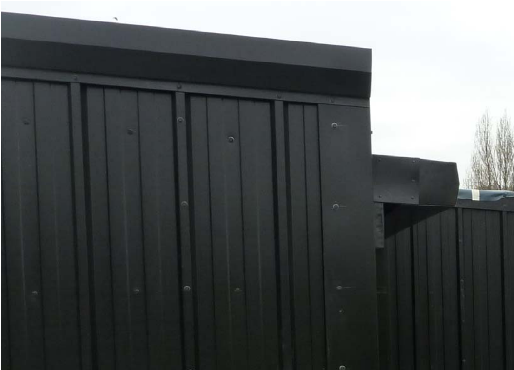
Fig.2 – Proposed trapezoidal black cladding on stair towers to be used for energy centre
