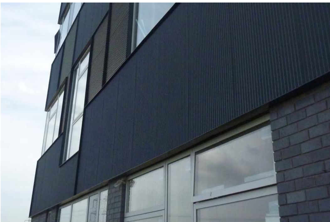
Fig.1 – Main school building brick & sinusoidal black cladding
