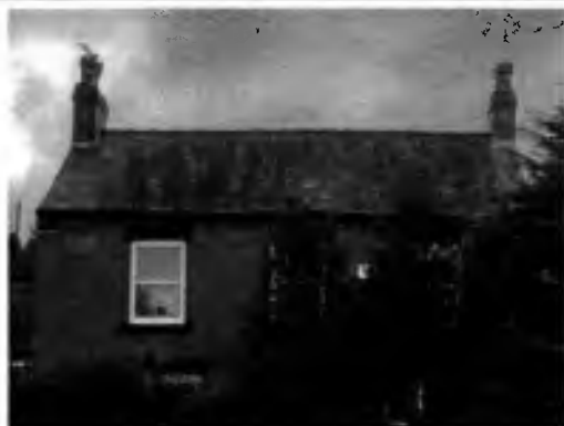
Photo 8: Front Roof Slope
