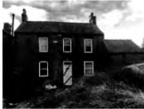
Photo 4: Rear of Property
