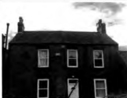
Photo 9: Rear Roof Slope
