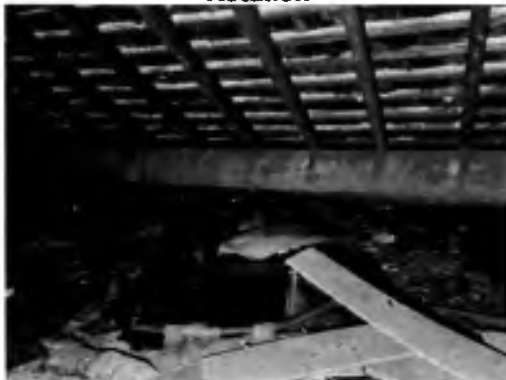
Photo 57: Rear Roof Slope
