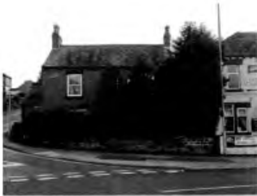
Photo 2: Front of Property
