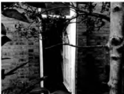
Photo 14: Tapered Infill to Front Door Frame
