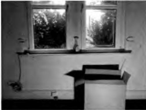
Photo 31: Front RHS Sloping Windowsill
