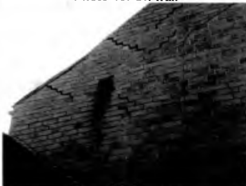
Photo 20: Cracking
