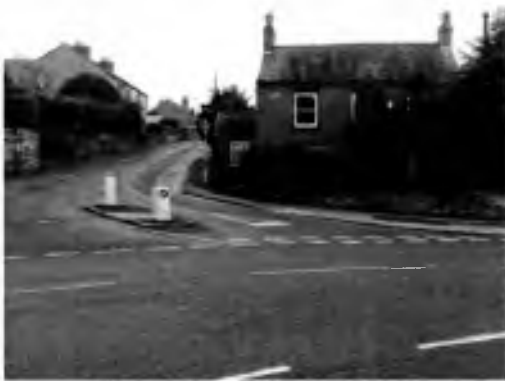
Photo 3: Front of Property
