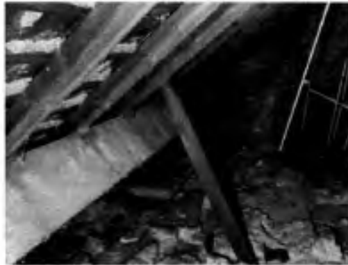
Photo 56: Front Roof Slope
