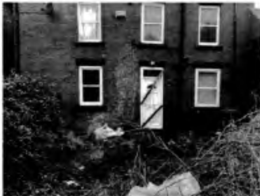
Photo 6: Roof and Foul Drainage to Rear
