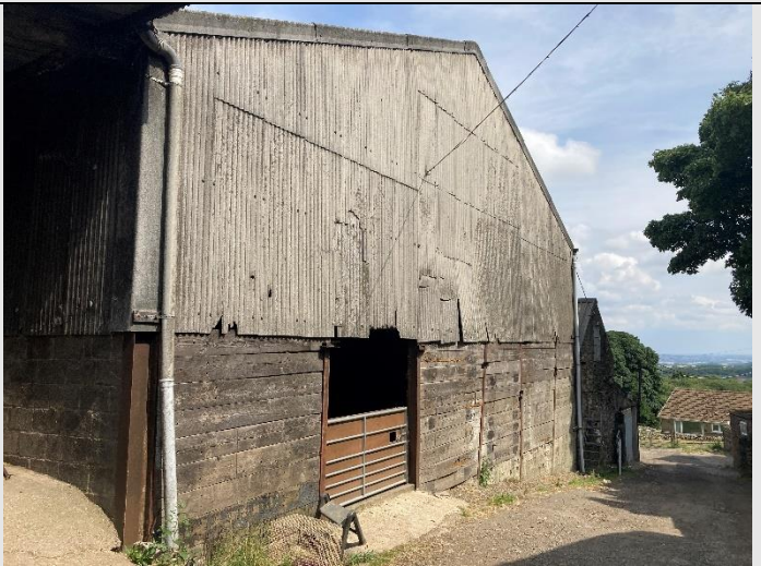
Figure 11. South eastern elevation of Building 2.
