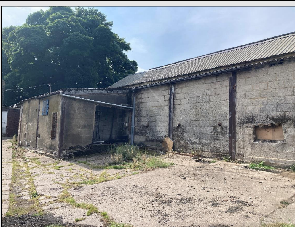
Figure 3. Area of hardstanding adjacent to building 6.
