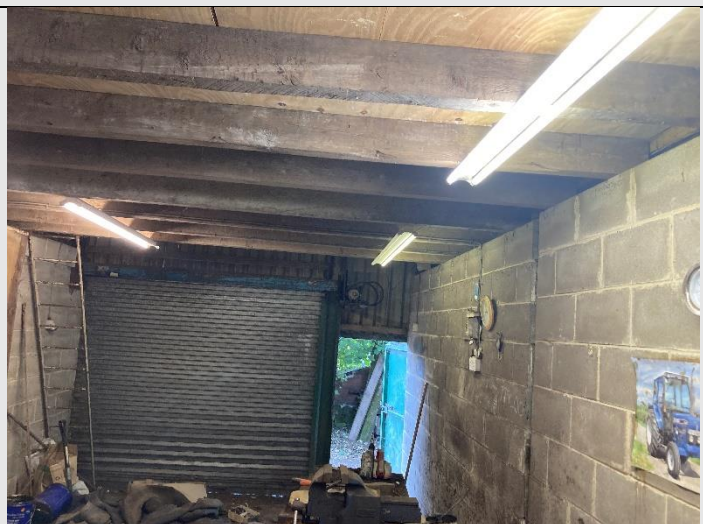
Figure 27. Interior of Building 11.
