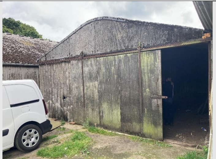
Figure 22. Northern elevation of Building 9.
