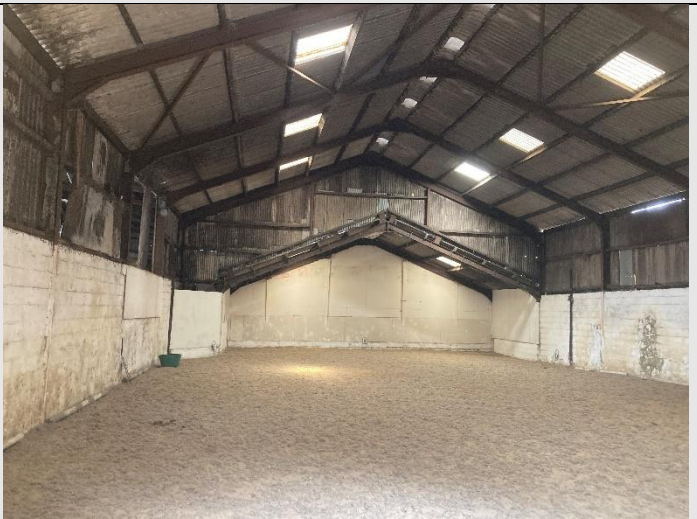
Figure 12. Interior of Building 2.
