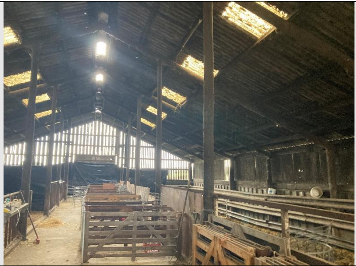
Figure 25. Interior of Building 10.
