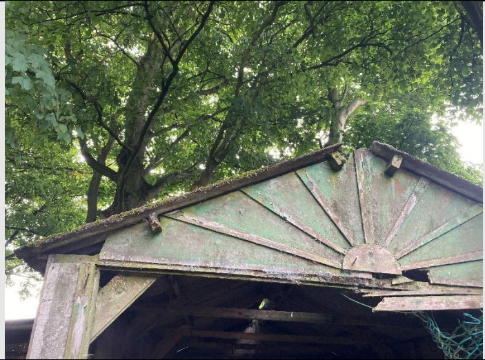
Figure 28. Northern elevation of Building 12.
