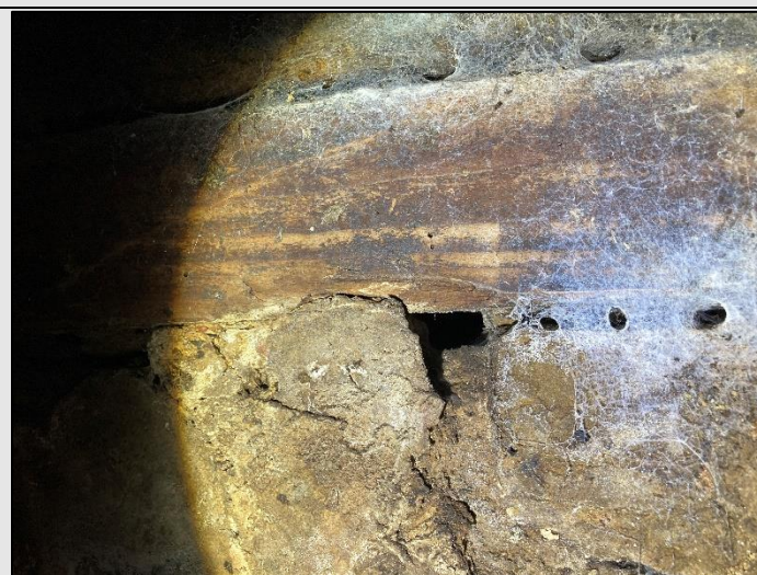
Figure 9. Internal crevices with hibernation suitability within Building 1.
