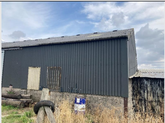
Figure 17. western elevation of Building 6.
