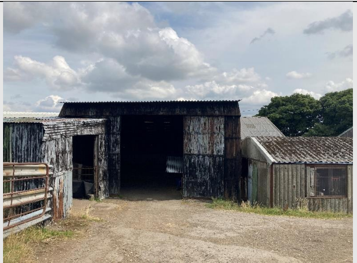
Figure 15. Western elevation of Building 5.
