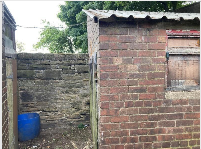
Figure 31. Northern elevation of Building 13.
