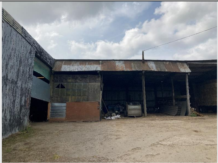
Figure 20. Northern elevation of Building 8.
