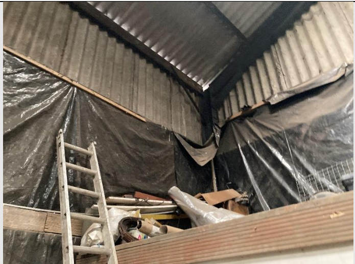
Figure 16. Interior of Building 5.
