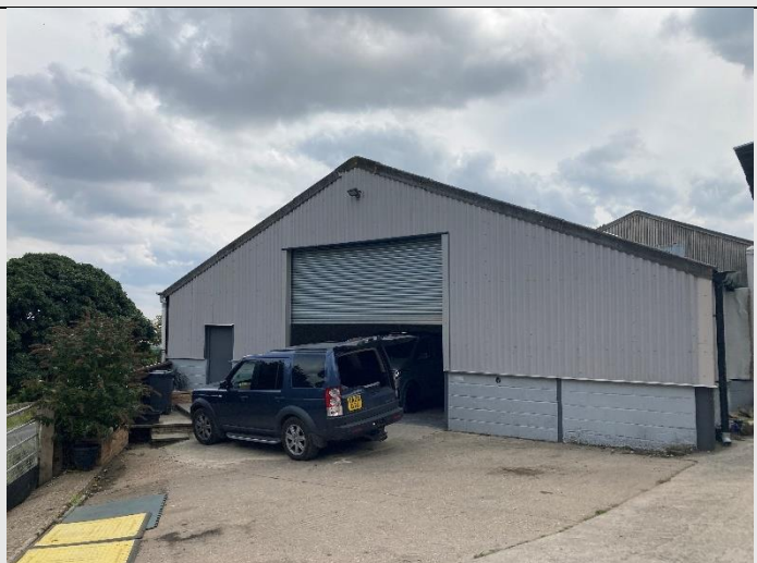
Figure 18. Northern elevation of Building 7.
