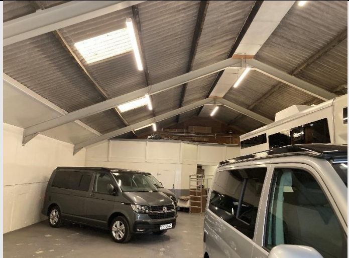
Figure 19. Interior of Building 7.
