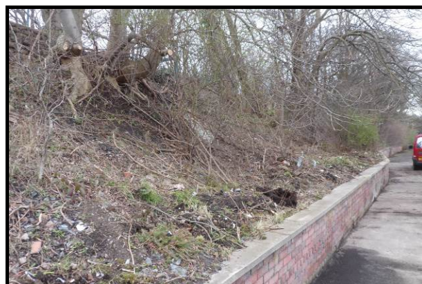
Figure 10. Disused railway embankment.
