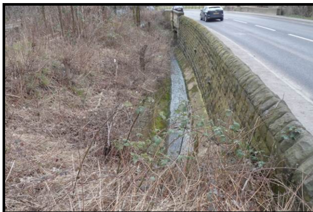
Figure 14. Culvert in Southern corner of site leading into River Dove.
