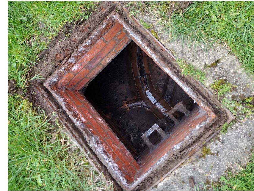
Existing Inspection Chamber 1
