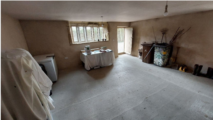
Ground floor room south side, there is a sand cement render to all walls and plasterboard to the ceiling and sand cement screed to the floors
