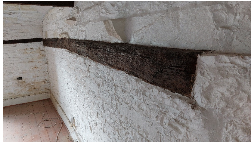
The original stone wall plate is visible in parts where the roof was raised.
