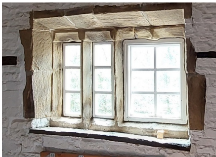
stone surround to first floor window
