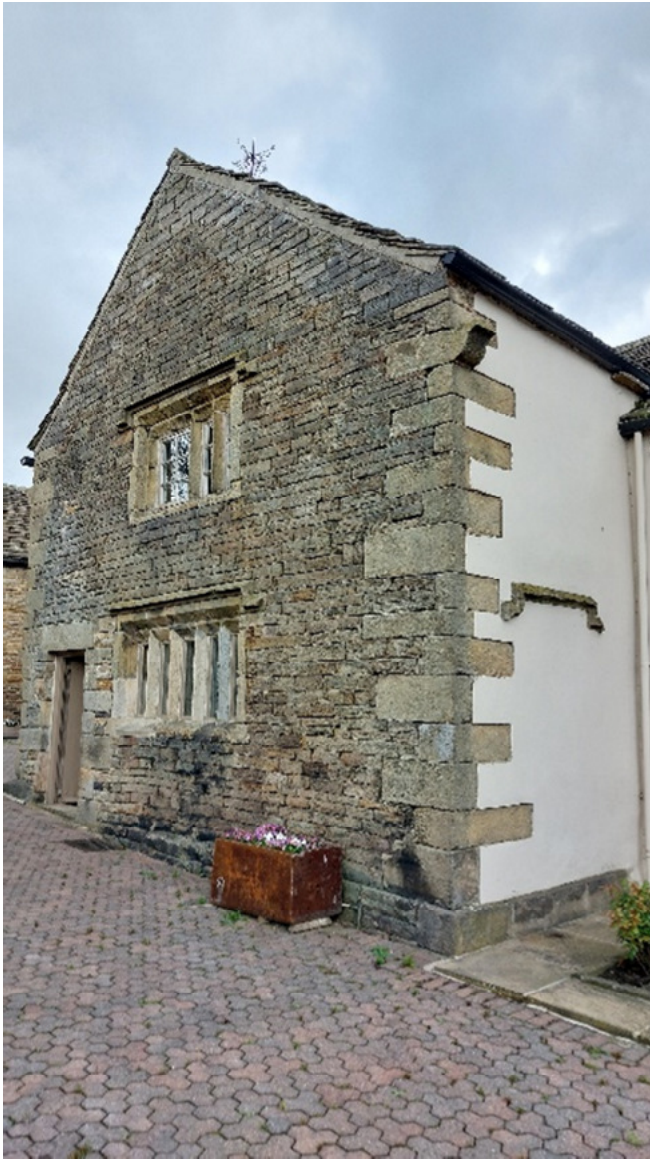
The west wing front (south) elevation, the roof has been raised at some point in its history by approximately 500mm as can be seen from the Kneelers and slight change in stone to the gable
