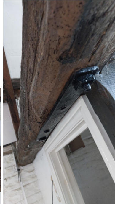
Steel plate to truss
