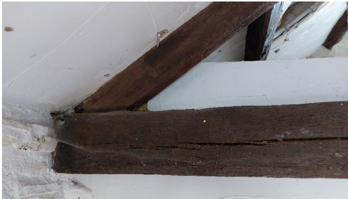
Truss to wall connection
