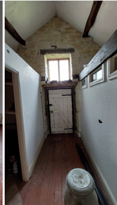
Modern plasterboard partitioning
