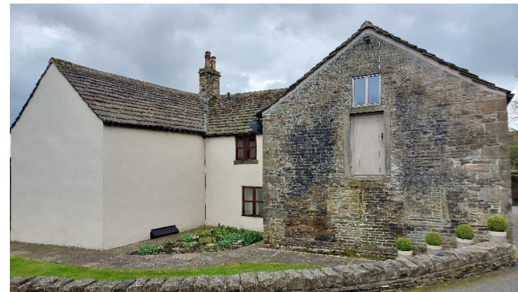
Rear (north elevations)
