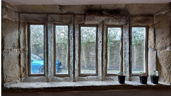
Kitchen window, render to be finished with a raked detail to the edge of the stone surround.
