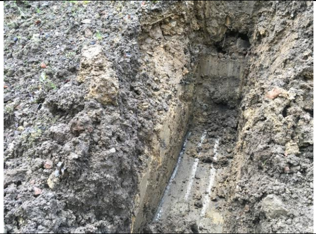
General trial pit excavations
