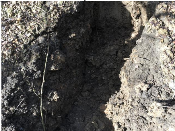
General trial pit excavations
