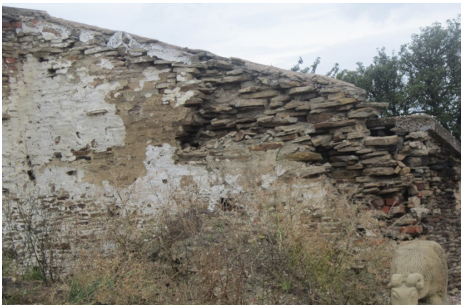
Outbuilding rear wall in poor state of repair
