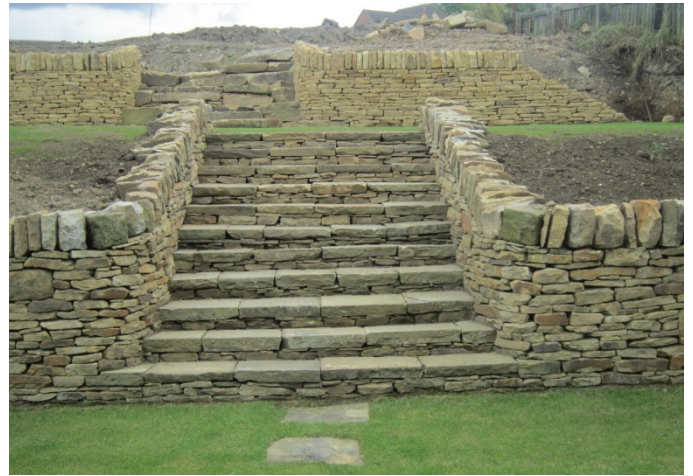
Dry Stone walling on the development
