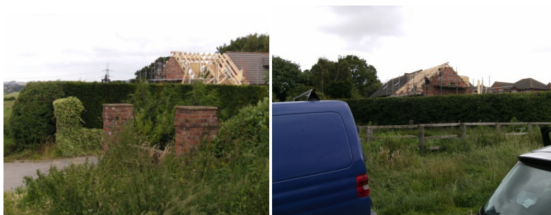
Extension to Surrounding Buildings
