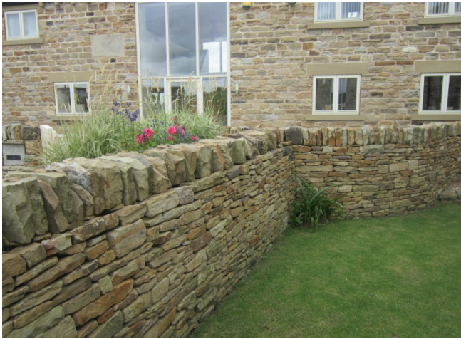
Dry Stone walling on the development
