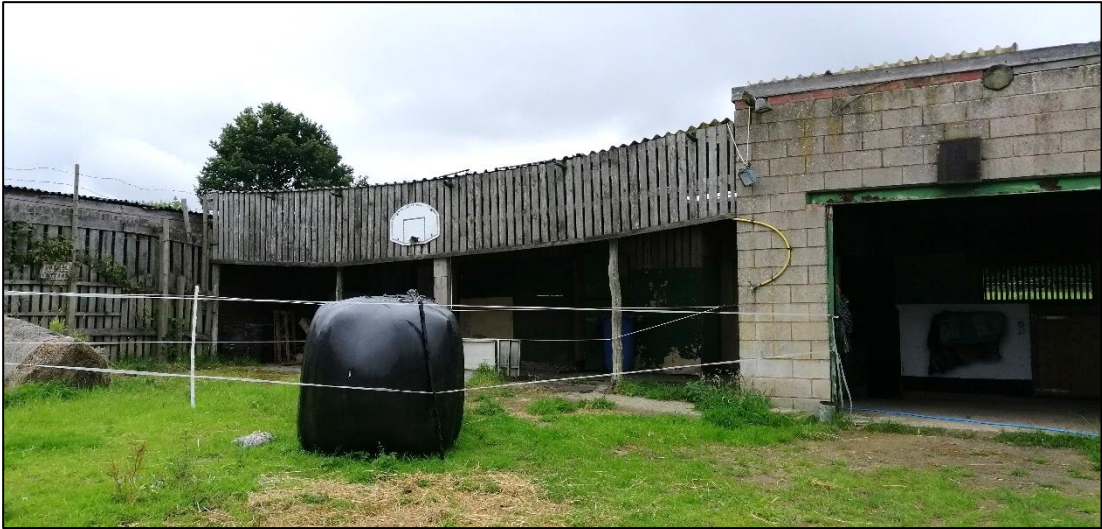
Plate 3. North end of B1 and adjoining B3
