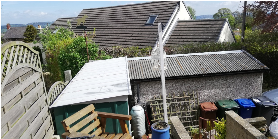
Pebble dash flat roof prefab garage and view from the existing terrace
