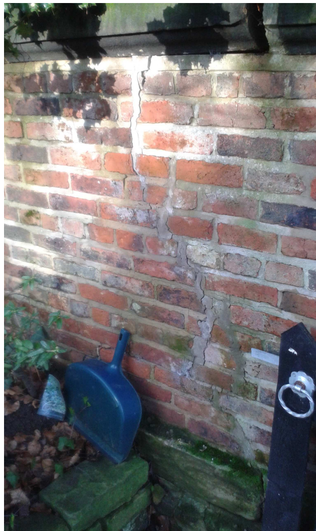
Photograph 2: Crack in north side of Grade 2 listed wall (left image). Crack in south side of Grade 2 listed wall with historical repair work (right image).
