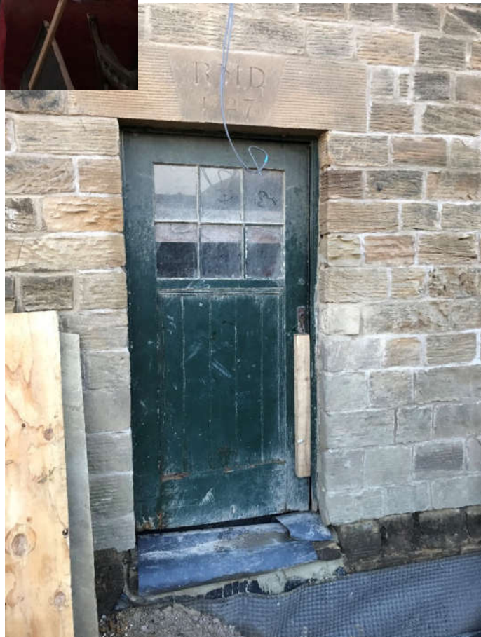
Existing Rear Door D3
