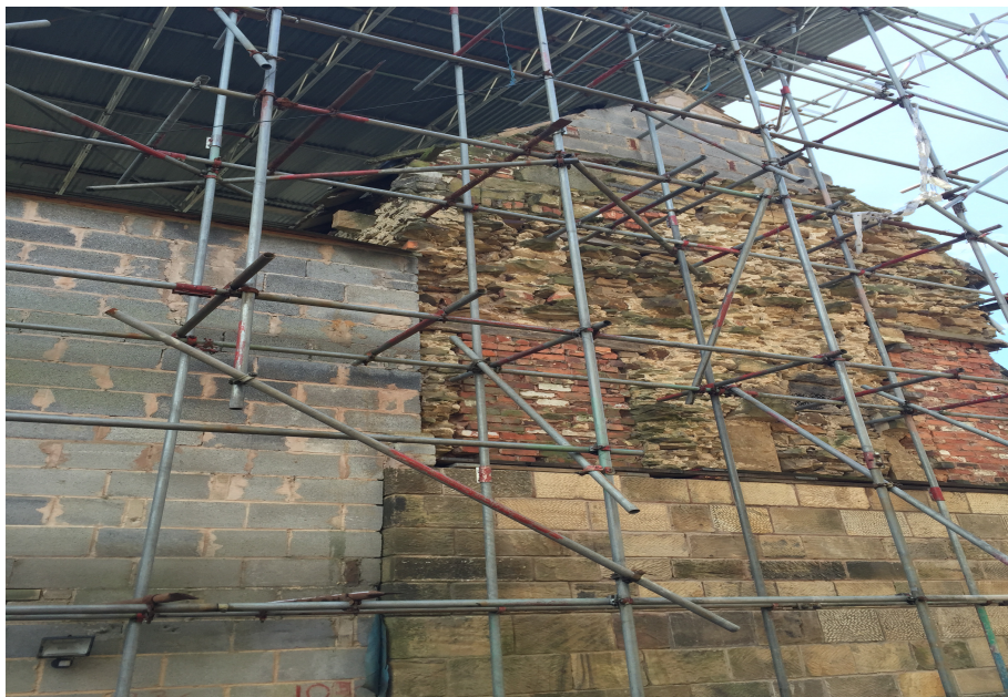
Photograph A – View of Wall
