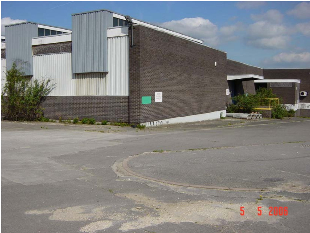
Plate 1 – Centre of Site facing north.
