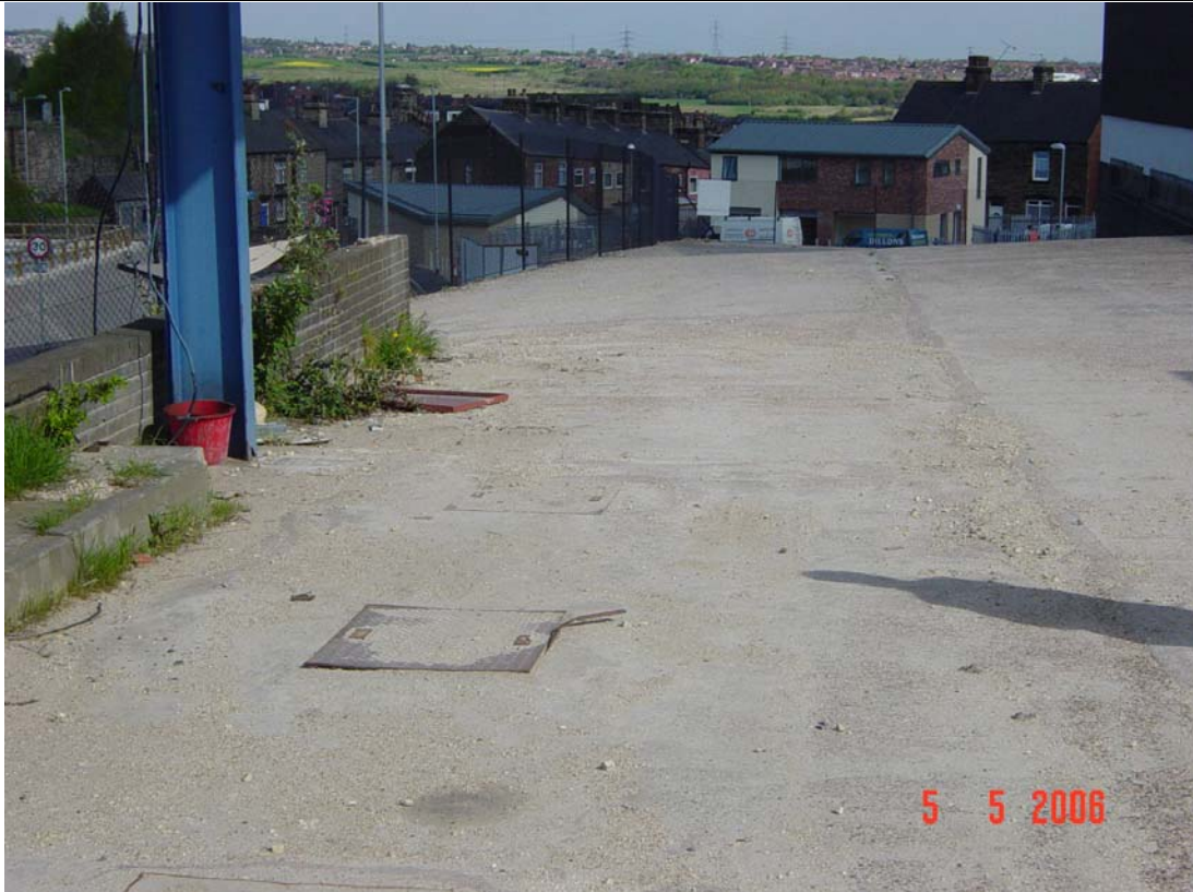
Plate 7 – West of the site between central building and perimeter with bus depot.
