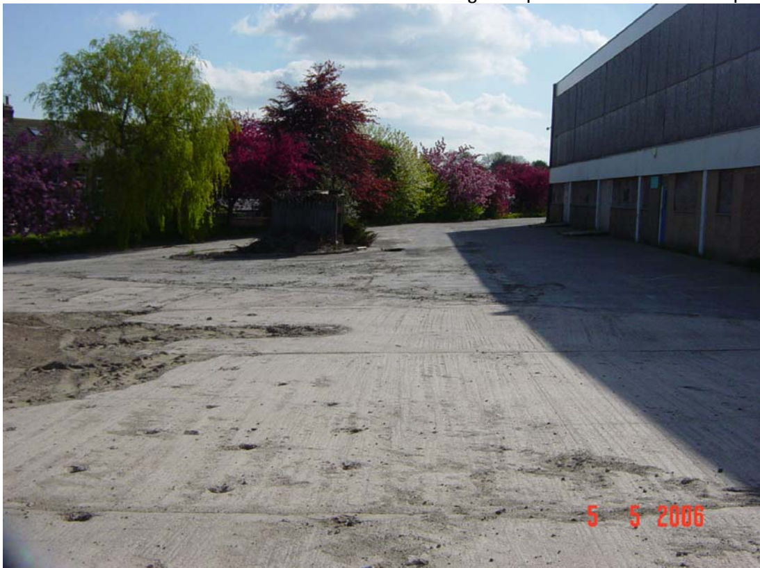
Plate 8 – North of the site behind central building viewing east.
