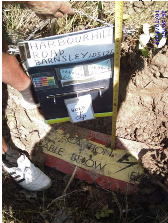
Plate 15 – Inspection Pit 4 where services were less than 0.50m from ground level.
