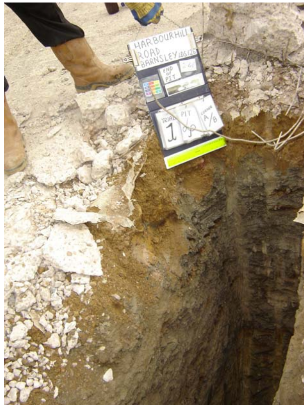
Plate 24 – Near surface rockhead Trial Pit 14. The pit was complete at 2.40m bgL.
