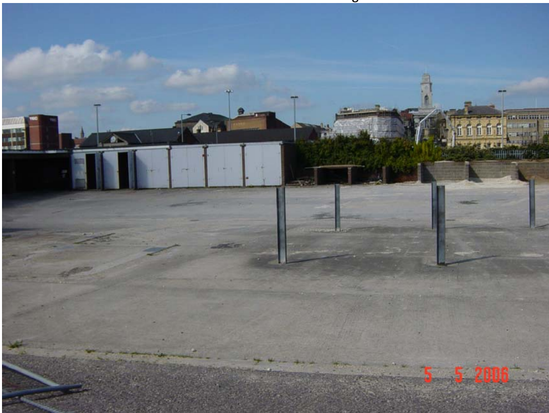
Plate 4- Derelict buildings in the south of the site.
