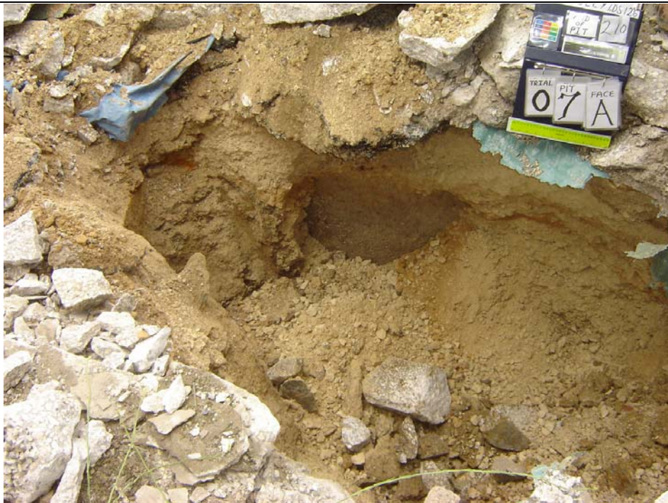
Plate 17 – Drain chamber unearthed at the side of face A Trial Pit 7 The area was unfilled with pavement material.
