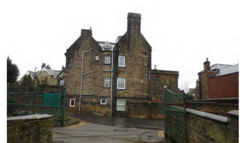
Image 4; Access from site onto Cockerham Lane showing neighbouring 2 and 3 storey Victorian housing.
