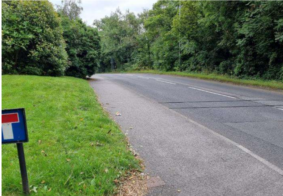
Photo 1: Footway on Keresforth Road
