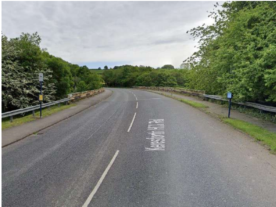
Figure 9: Existing Bus Stops on Keresforth Hill Road
