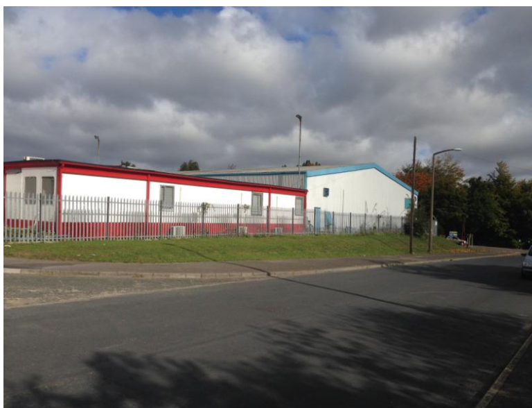
Figure 4 – View to the right hand side of the site entrance
