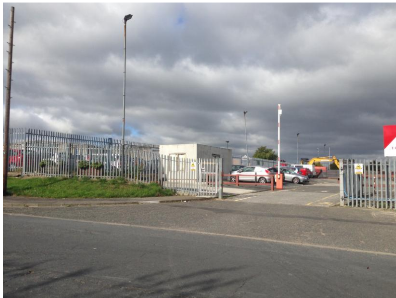
Figure 3 – View across site entrance including the gate house
