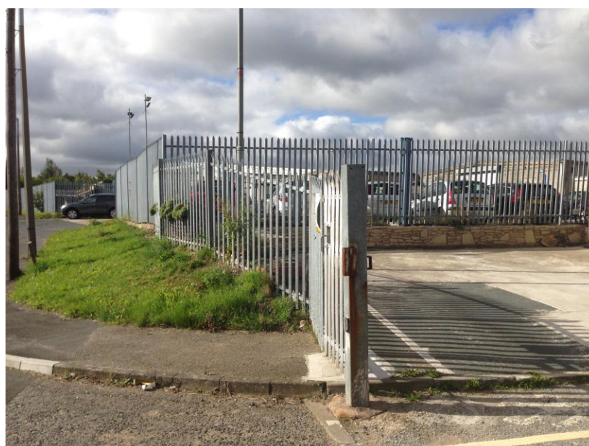
Figure 6 – View of existing gate on site
