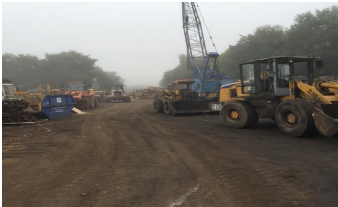
Figure 2 View looking southwards along the site.
