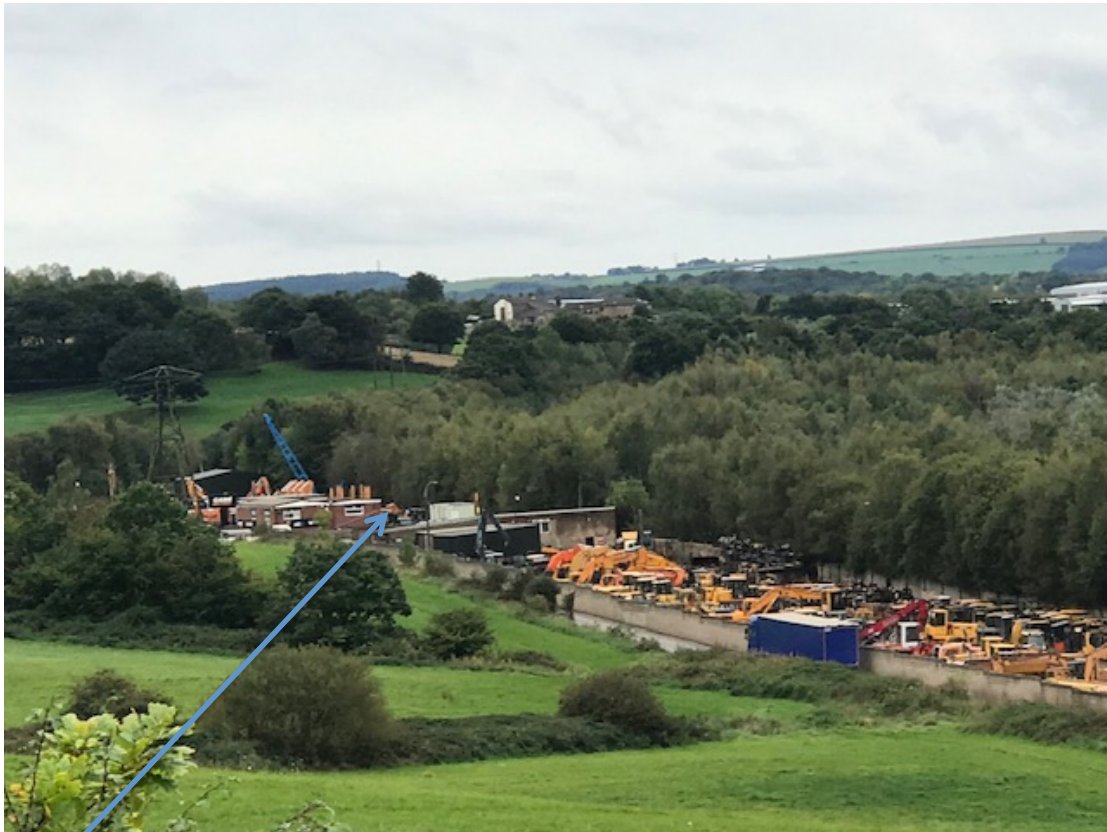
Figure 3View of industrial premises from elevated position to the east
