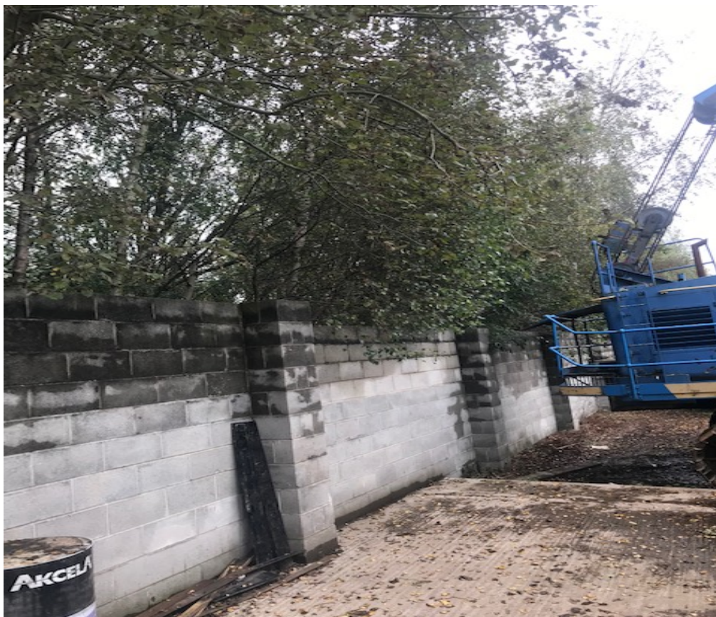
Figure 5 Overhanging trees on boundary
