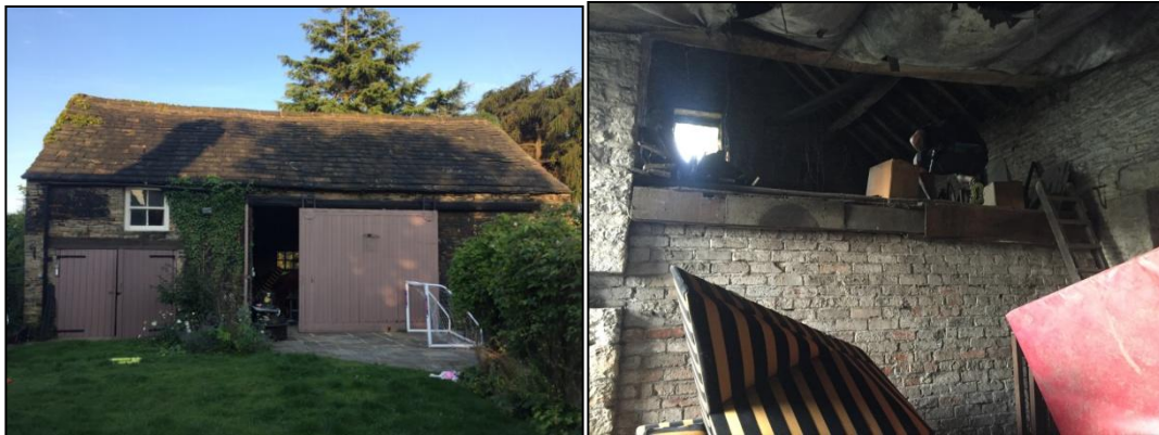
Figure 3. View of surveyed building.
