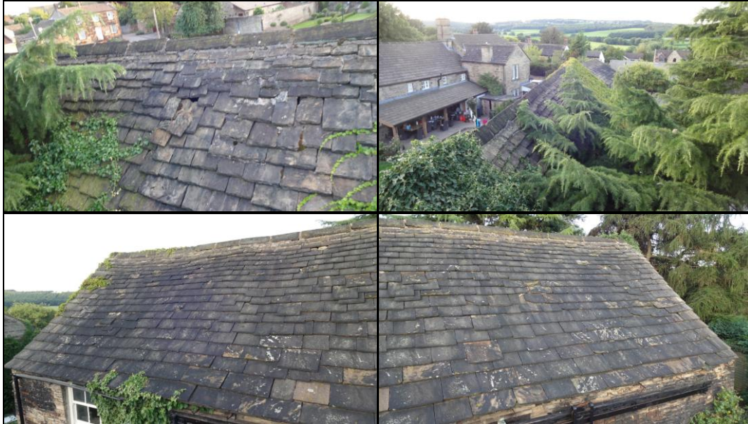
Figure 7. View of roof.
