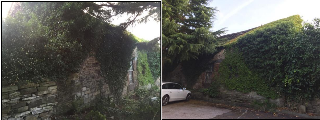
Figure 5. View of rear of building.
