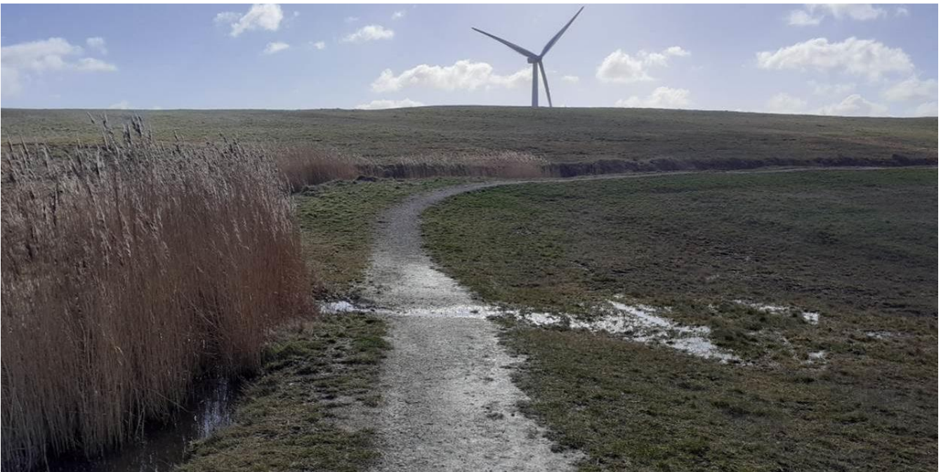
Plate 3: View of overflow feeding Orchid Receptor Area 1, due to be 'formalised' and made permanent.
