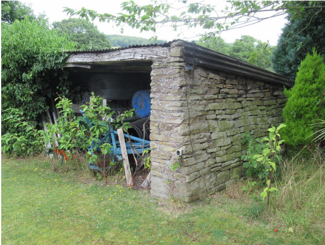
Photograph 3 – Southern elevation of the building.
