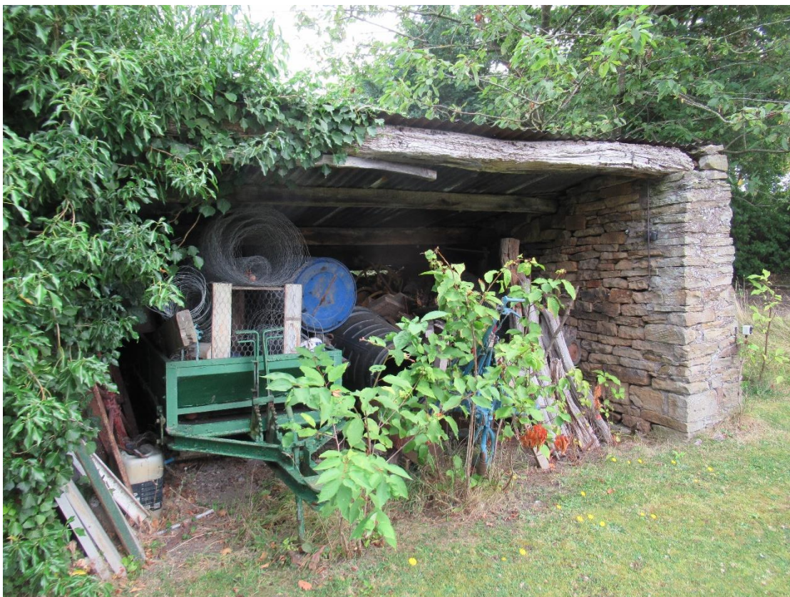
Photograph 2 – Western elevation of the building, south of the dividing wall.
