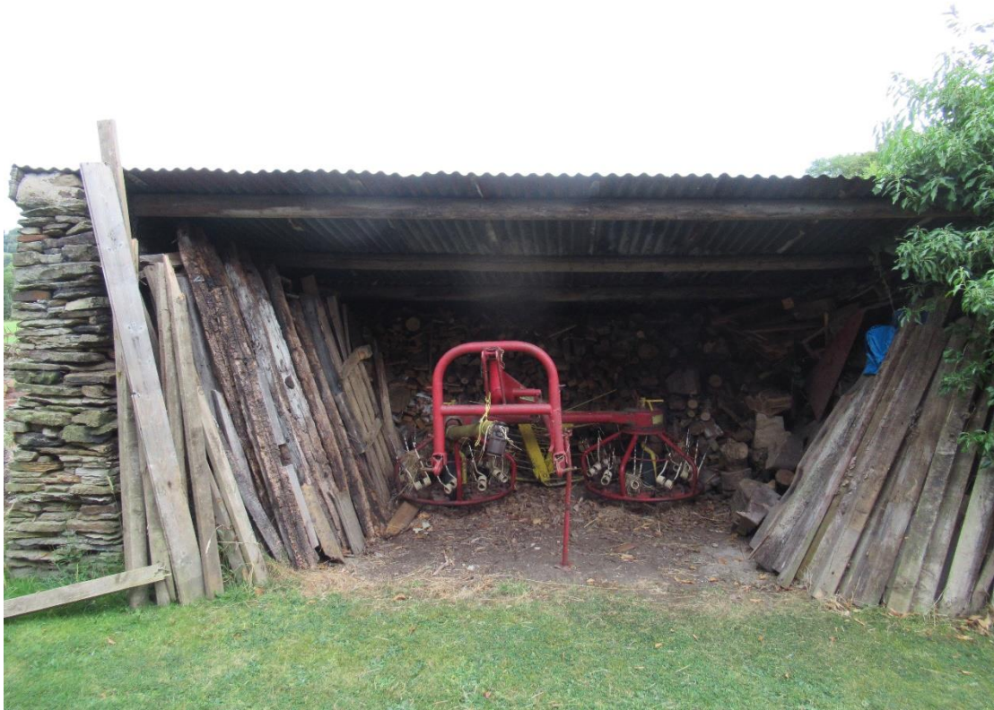
Photograph 1 – Western elevation of the building north of the dividing wall.
