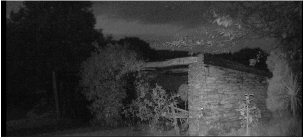
Surveyor position 1 – North-east of the building on 19 th August 2024.
