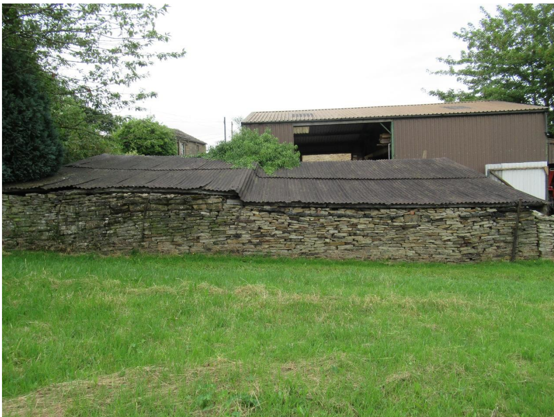
Photograph 4 – Eastern elevation of the building.
