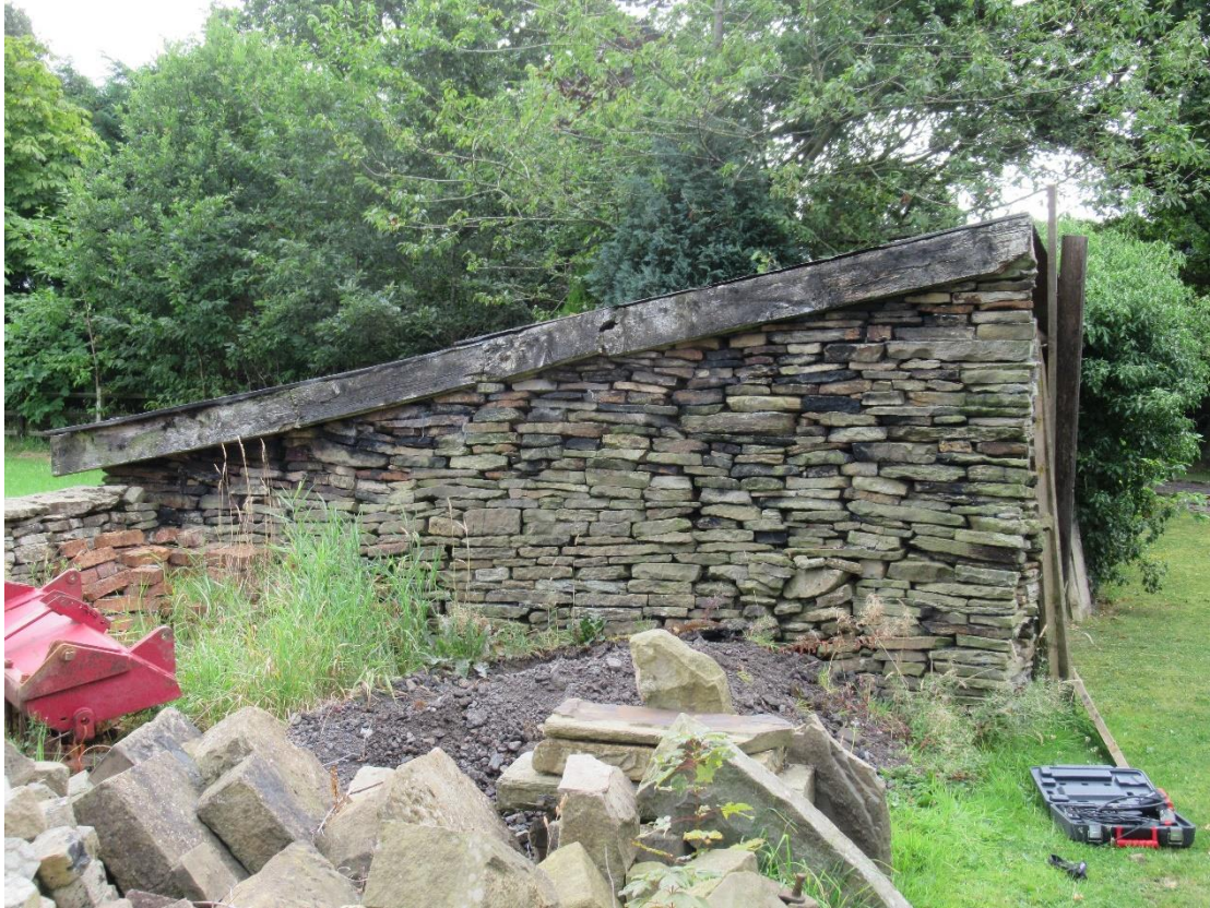
Photograph 5 – Northern elevation of the building.
