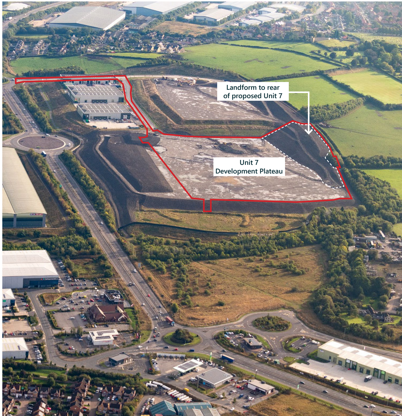
Fig. 1 Aerial view of Site showing extent of RM Application and location of constructed landform
