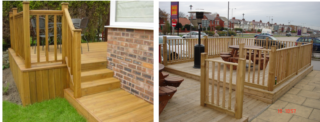
PHOTOGRAPHS SHOWING TYPICAL RAISED DECKING & BALUSTRADE
