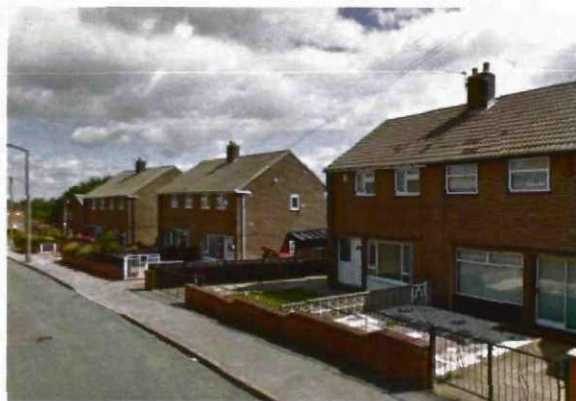
1. View of houses 70 & 72 to be demolished off Cypress Road.
