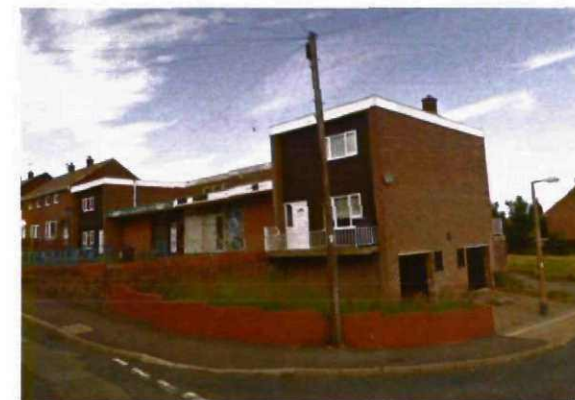
5. Existing units off Farm Road to be demolished.
