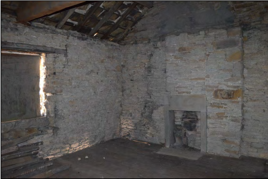
Figure 18: View of first floor room F3 , looking east
