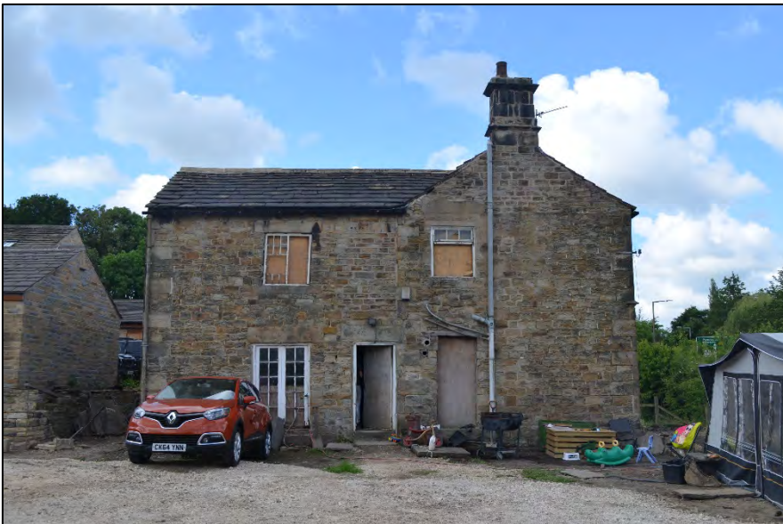
Figure 8: View of the south-east elevation of Bank House
