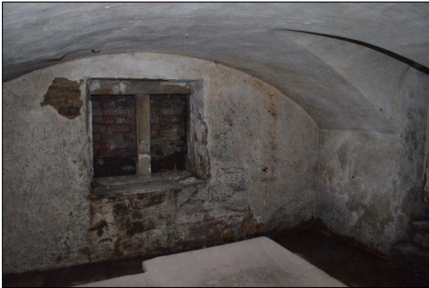
Figure 15: View of cellar room C1 , looking north.
