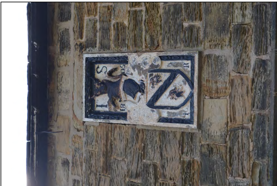
Figure 12: View of the coat of arms on the north-east elevation
