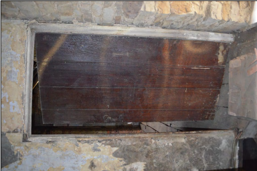
Figure 22: View of plank and ledged door to F1 , looking north-east
