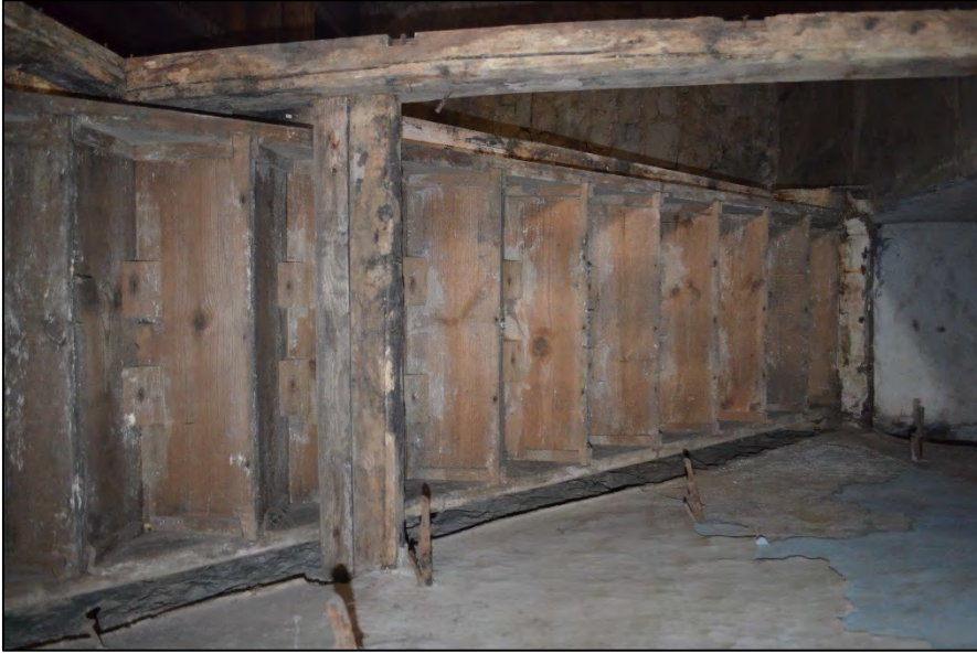
Figure 23: View of the underside of the stairs in G1 , noting replaced risers.
