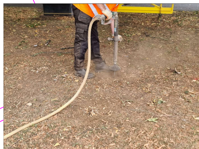
Figure 2: Photo of Air excavation in action © Selwyn Trees:
