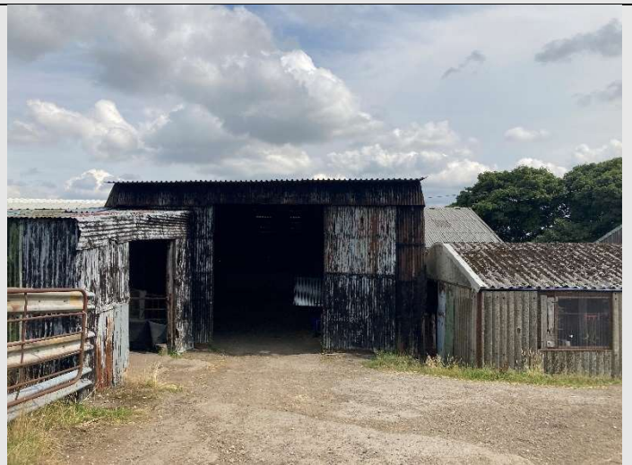
Figure 15. Western elevation of Building 5.
