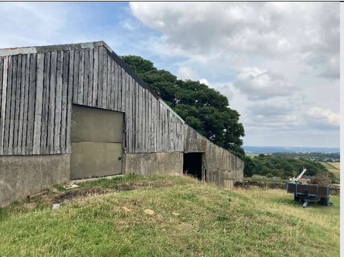
Figure 24. Southern elevation of Building 10.
