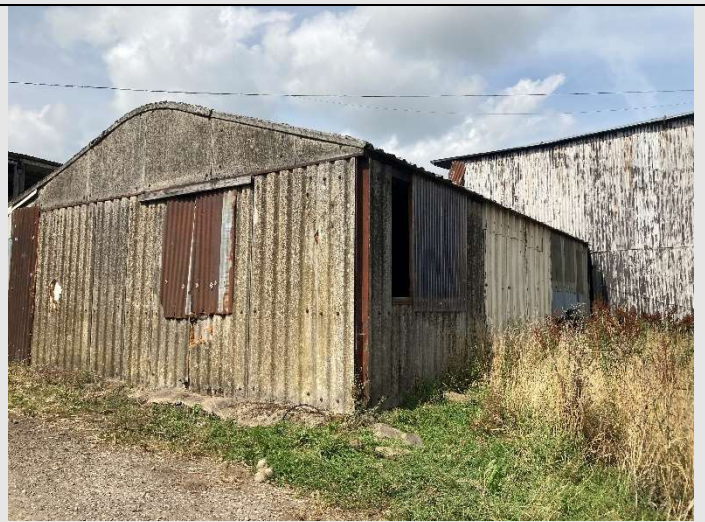
Figure 14. Southern elevation of Building 4.
