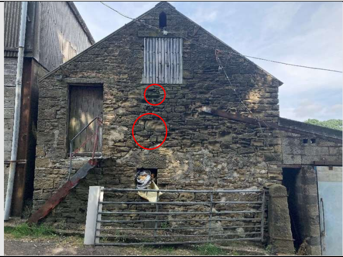
Figure 7. Southern elevation of Building 1 showing two storey stone wall. Gaps in mortar providing roosting potential.
