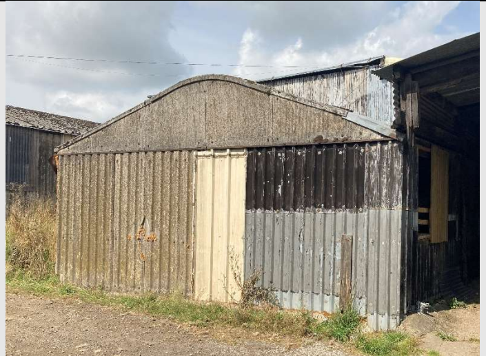
Figure 13. Southern elevation of Building 3.
