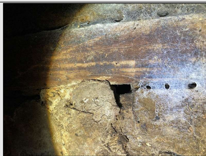
Figure 9. Internal crevices with hibernation suitability within Building 1.
