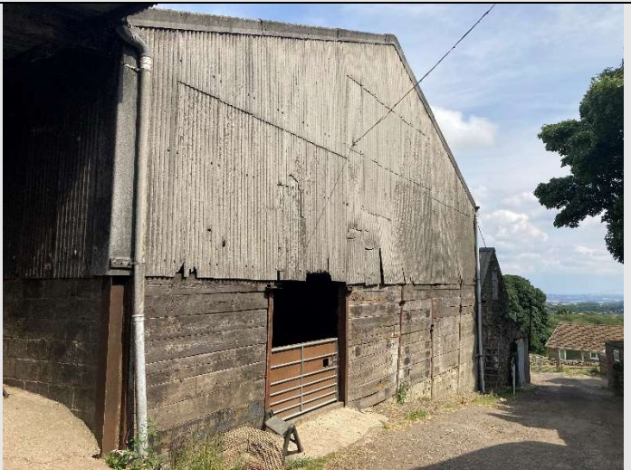
Figure 11. South eastern elevation of Building 2.
