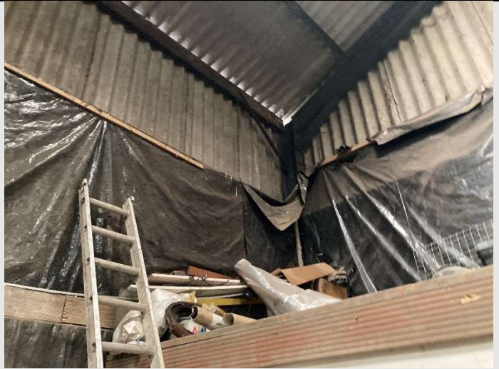
Figure 16. Interior of Building 5.
