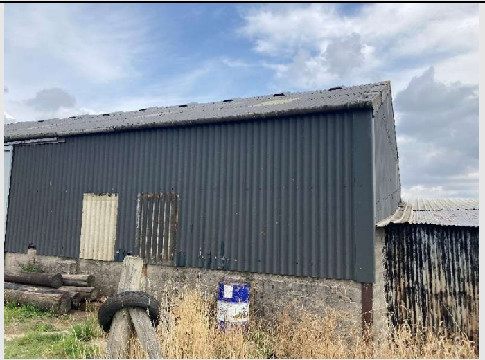
Figure 17. western elevation of Building 6.
