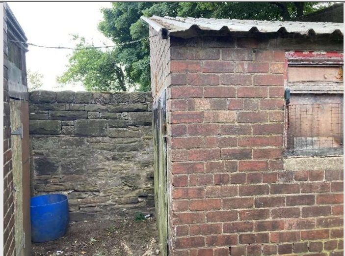
Figure 31. Northern elevation of Building 13.
