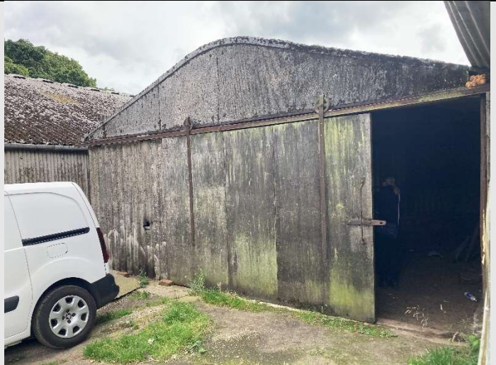
Figure 22. Northern elevation of Building 9.
