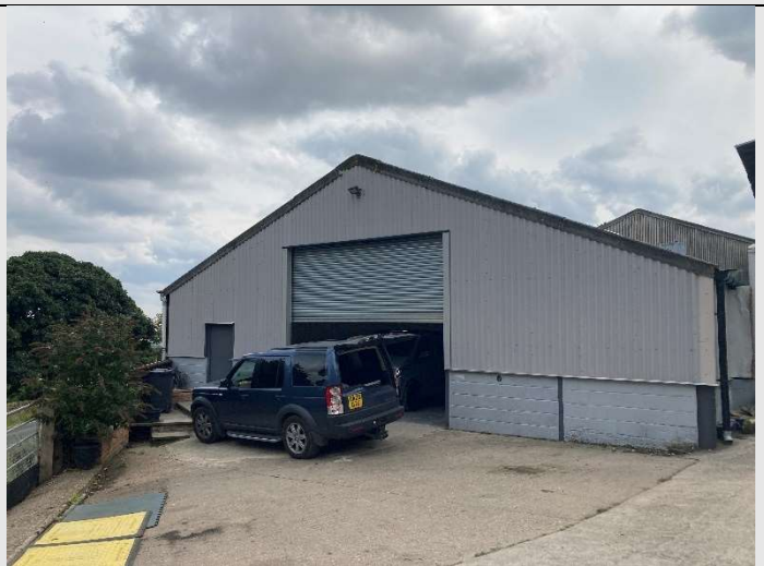
Figure 18. Northern elevation of Building 7.
