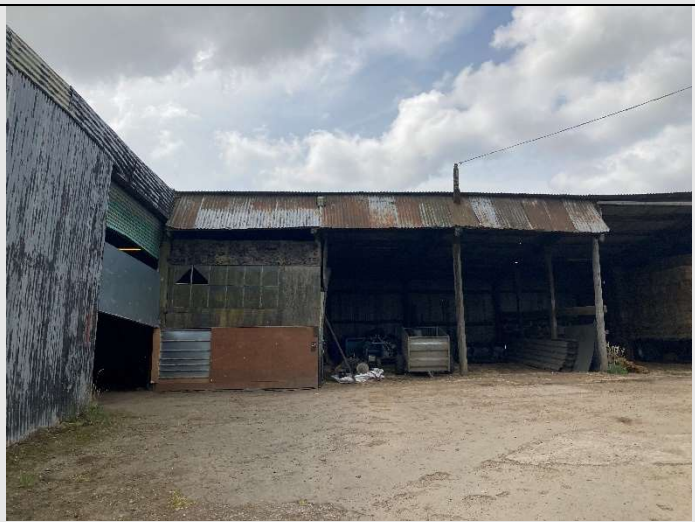
Figure 20. Northern elevation of Building 8.
