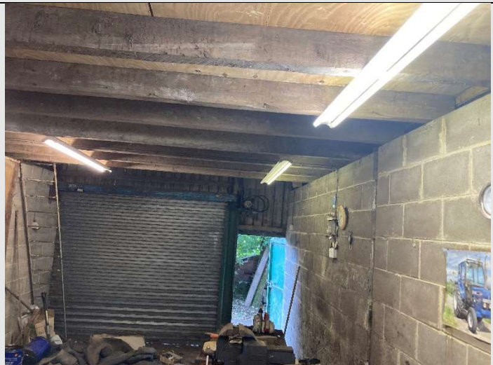
Figure 27. Interior of Building 11.
