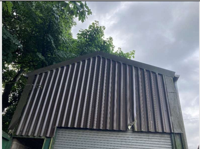
Figure 26. Eastern elevation of Building 11.
