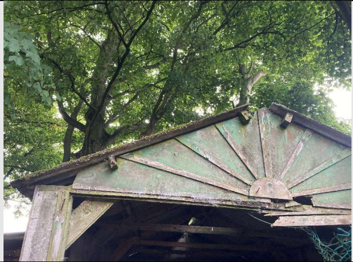
Figure 28. Northern elevation of Building 12.
