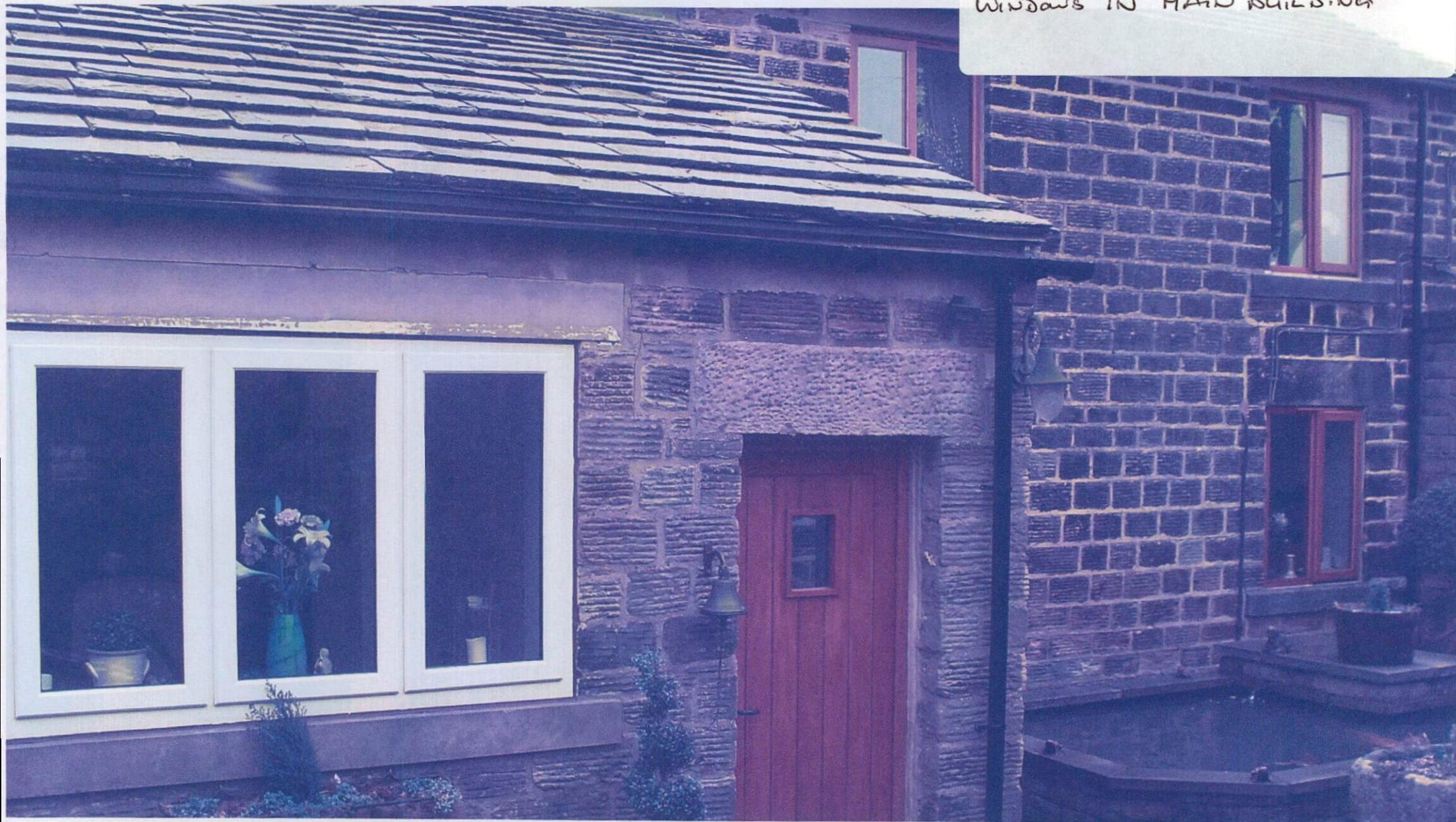
EAST FACING SHOWING ONE WINDOW AND HARDWOOD WINDOWS IN MAIN BUILDING
