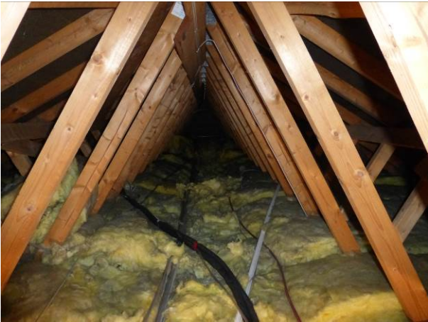
Fig. 7. Purchasing Sales – western roof void.
