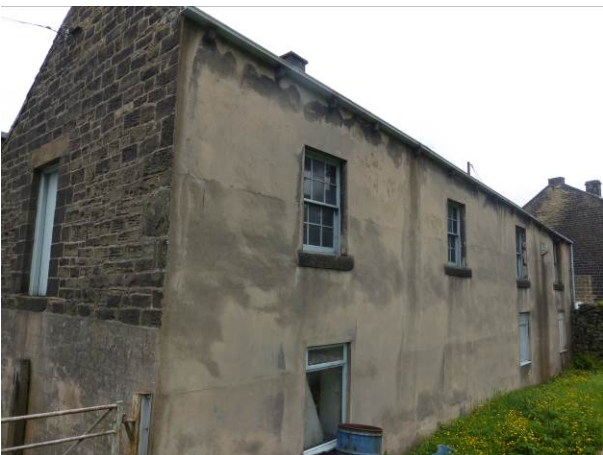
Fig. 5. Old Printing Store – north/east elevations.
