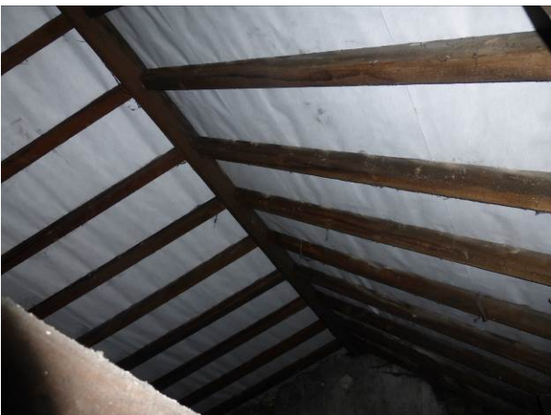
Fig. 11. Old Top Office – eastern roof void.
