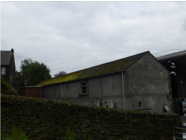
Fig. 9. Purchasing Sales – north/west elevations
