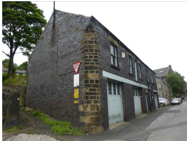
Fig. 4. Old Printing Store – south/west elevations.
