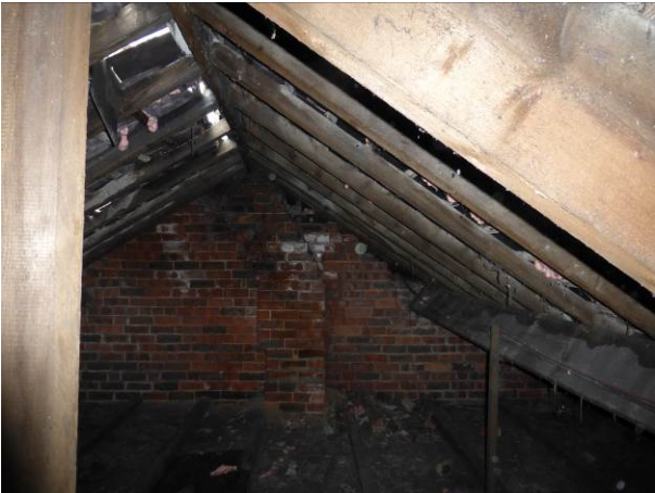
Fig. 1. Old Printing Store – roof void.
