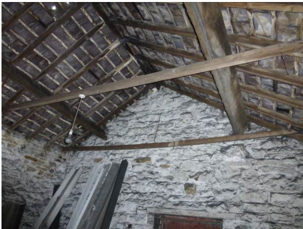
Fig. 3. Old Printing Store – open roof section.
