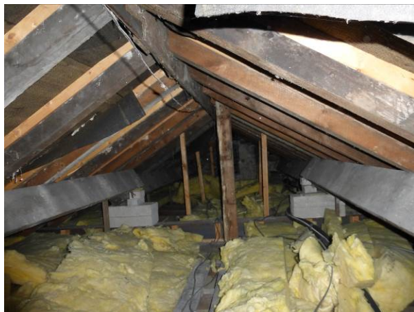
Fig. 6. Purchasing Sales – eastern roof void.
