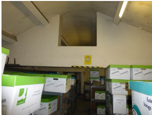
Fig. 10. Old Top Office – western roof void.
